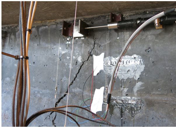
Crack propagation into composite slab at failure
