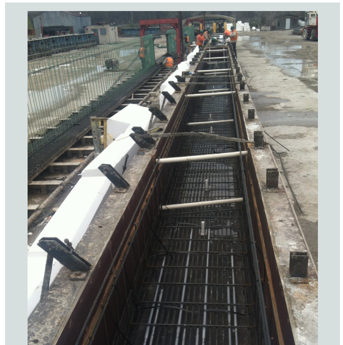
Figure 12. Reinforcement setup in a beam before concrete placement.
