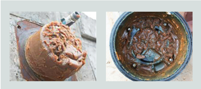
Figure 3. Anchor cap inspection (injection 4).
