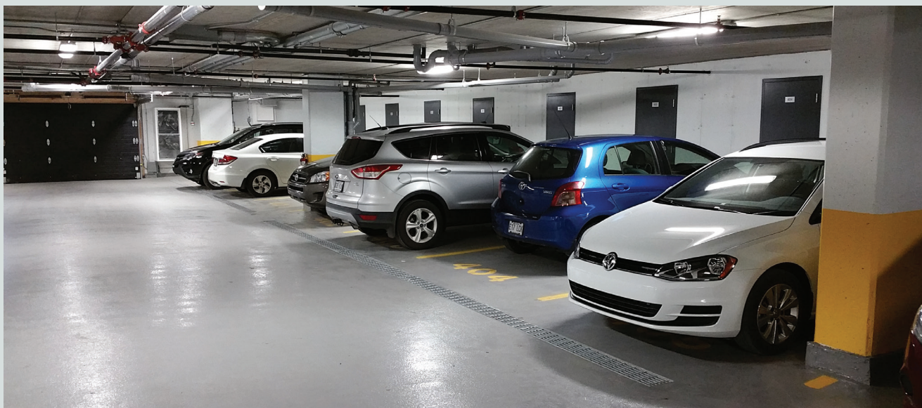
Figure 1. Top surface of a parking structure constructed with hollow-core slabs with drains inside the voids.
