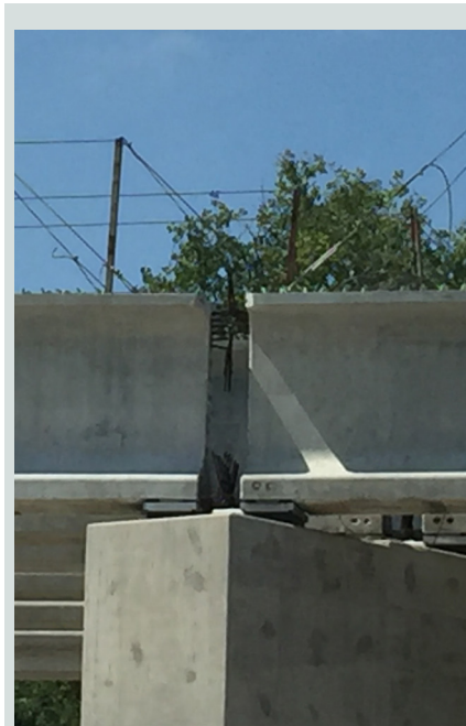
Figure 11. Bridge under construction near Des Moines, Iowa. Note the bent strands.
