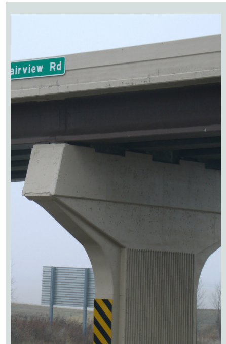
Figure 12. Fairview Road overpass over Interstate 80 in Omaha, Neb.
