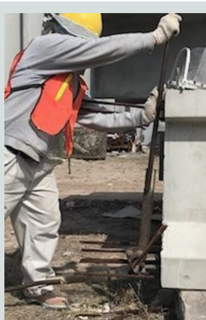
Figure 10. Strand bending at beam end. Courtesy of Coreslab Structures, Omaha, Neb.
