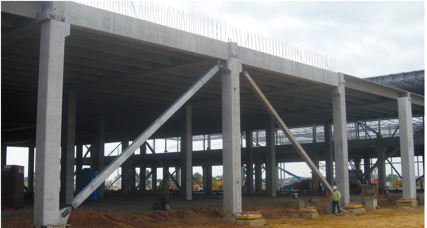
Typical buckling-restrained braced frame.
