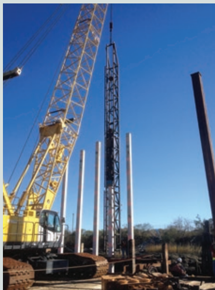
Figure 3. Pile driving operation (left) and extraction of piles through water jet stream applied at the bottom of the pile (right).
