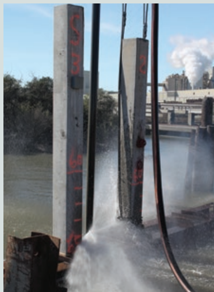
Figure 3. Pile driving operation (left) and extraction of piles through water jet stream applied at the bottom of the pile (right).
