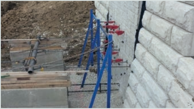
Instrumentation system showing steel frame with linear variable differential transformers attached
