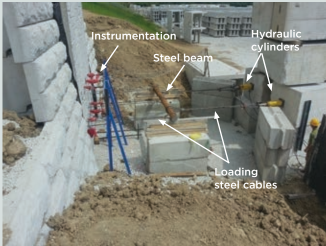
North view of setup
