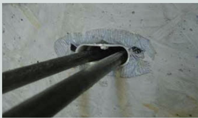
Figure 10. Posttensioned flange-to-flange connection before joint grouting.
