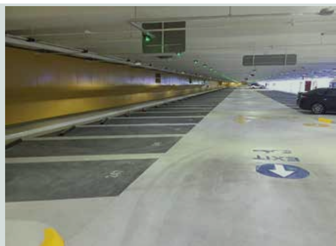
Figure 21. Inside view of a completed parking structure in Abu Dhabi, United Arab Emirates.
