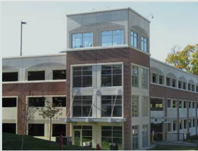
Figure 1. Precast concrete parking structure with exterior thin-brick load-bearing walls.
