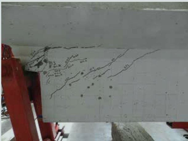
Diagonal tension cracking within the nib
