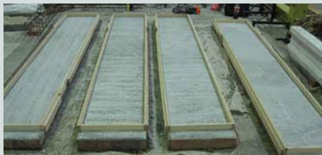
Before casting the topping
