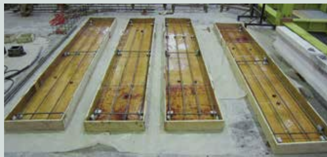
Before casting the substrate
