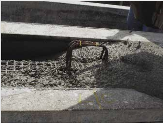
During concrete casting
