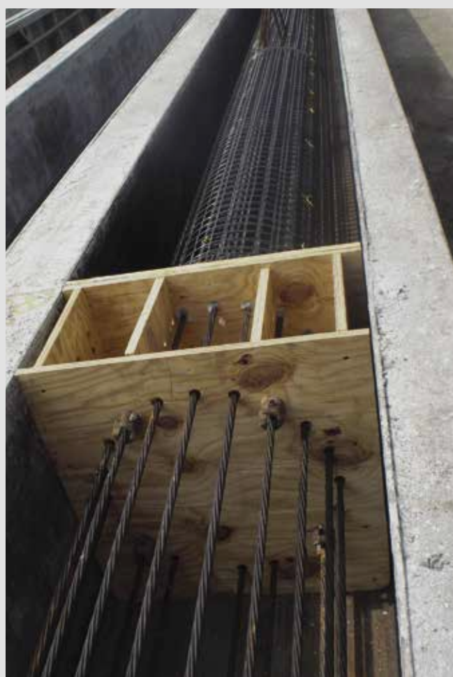
Figure 13. Pile with carbon-fiber-reinforced polymer grid before concrete casting.
