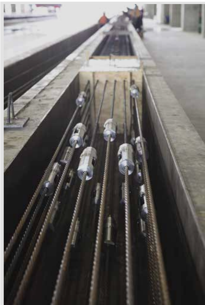
Figure 4. The couplers were staggered to prevent interference during stressing. The steel strands are in the foreground and the carbon-fiber-composite cable (CFCC) strands are in the background. Couplers connect the steel strands to the CFCC strands.
