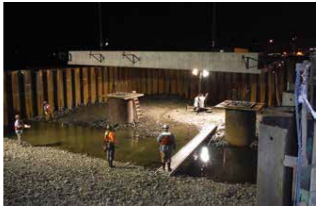
The precast concrete portion of the crossbeam is set in place on the precast concrete columns. The intermediate piers were constructed during the second fish window (summer 2014) within the wetted perimeter of the Cedar River. The use of precast concrete accelerated construction, allowing it to be completed during the allotted work window. Courtesy of Greg Banks.
