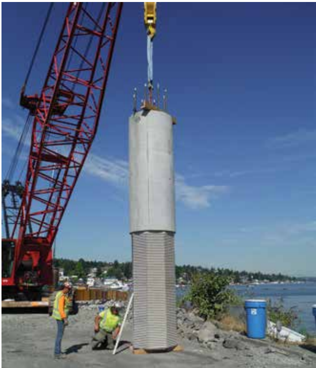
The intermediate pier column is about to be lifted and set into position. The corrugated portion of the column was embedded into the cast-in-place drilled shaft. Courtesy of Greg Banks.
