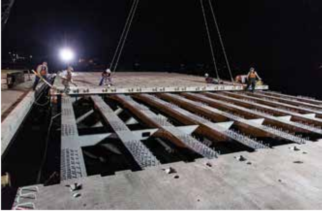
The full-depth precast concrete deck panels were erected on top of the steel plate girders. Due to proximity to the runway, this work was done at night to avoid interfering with operations at Renton Municipal Airport. Courtesy of Ramón Mariano, Jr.
