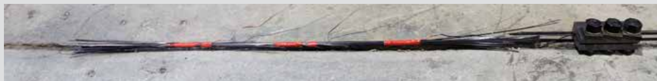
Figure 10. Fracture of carbon-fiber-reinforced polymer posttensioned rod.
