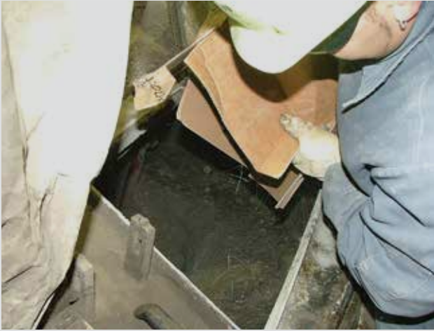
Concrete mixing with steel fiber
