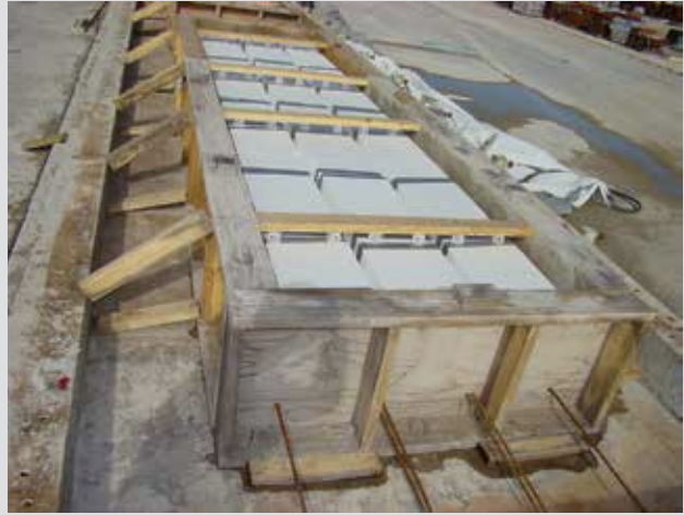
Preparation of formwork
