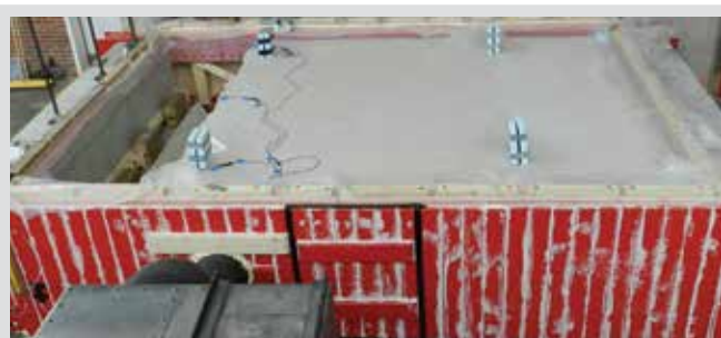
Figure 4. Typical failure of left flange cantilever.
