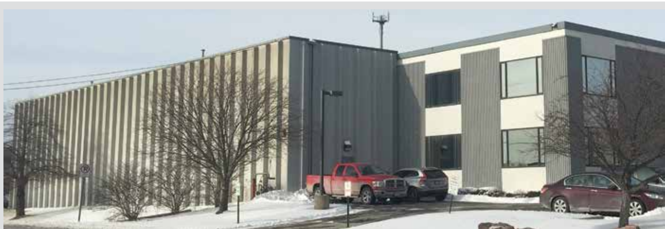
Figure 2. Example of the use of a double tee as a vertical load-bearing wall in an warehouse-office building in Omaha, Neb.
