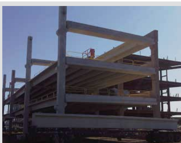
Figure 13. ConRAK Structure at Logan Airport in Boston, Mass., during erection with 60 ft (18.3 m) inverted-tee beam in foreground. Courtesy of Parsons Brinkerhoff and The Consulting Engineers Group Inc.
