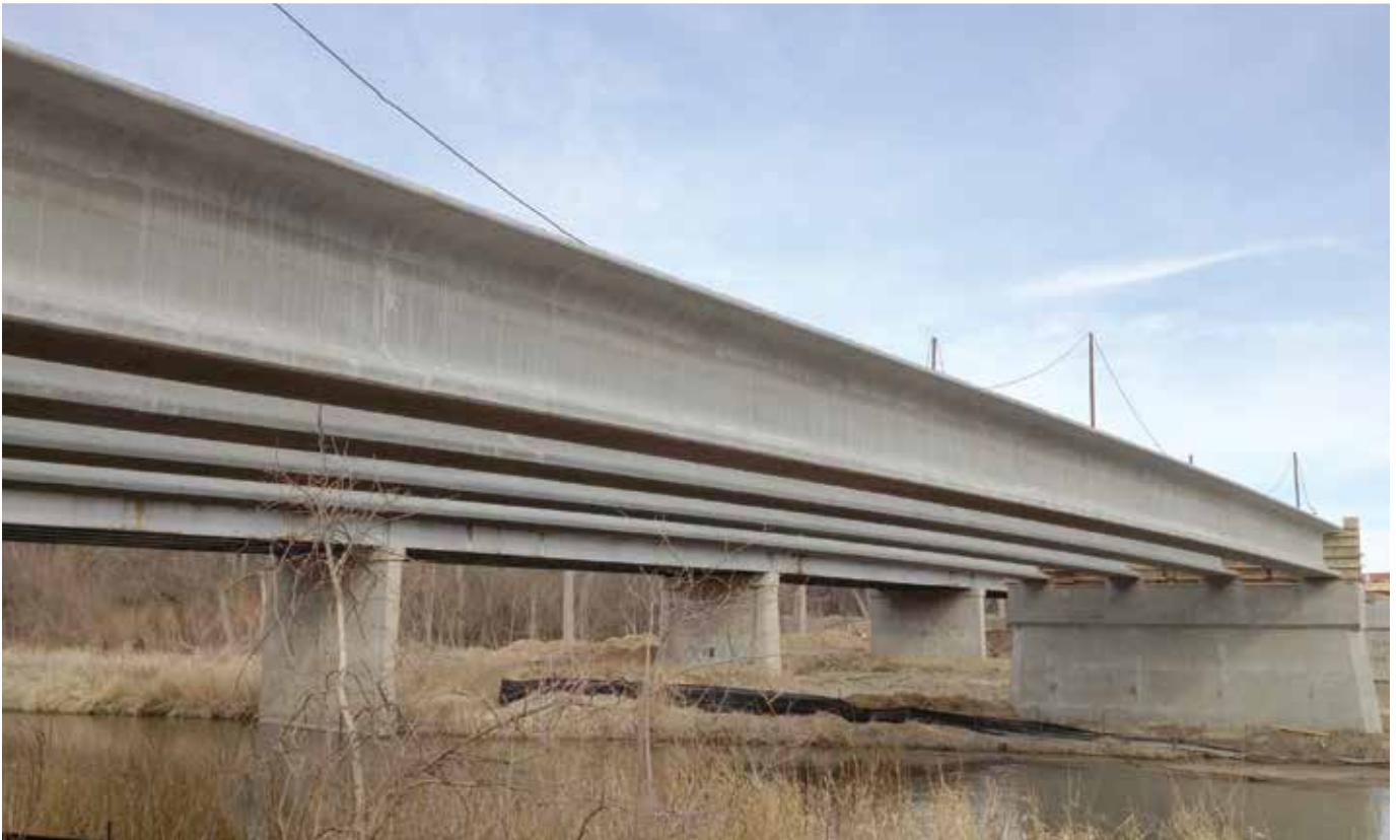
Figure 9. Girders directly before deck forming.
