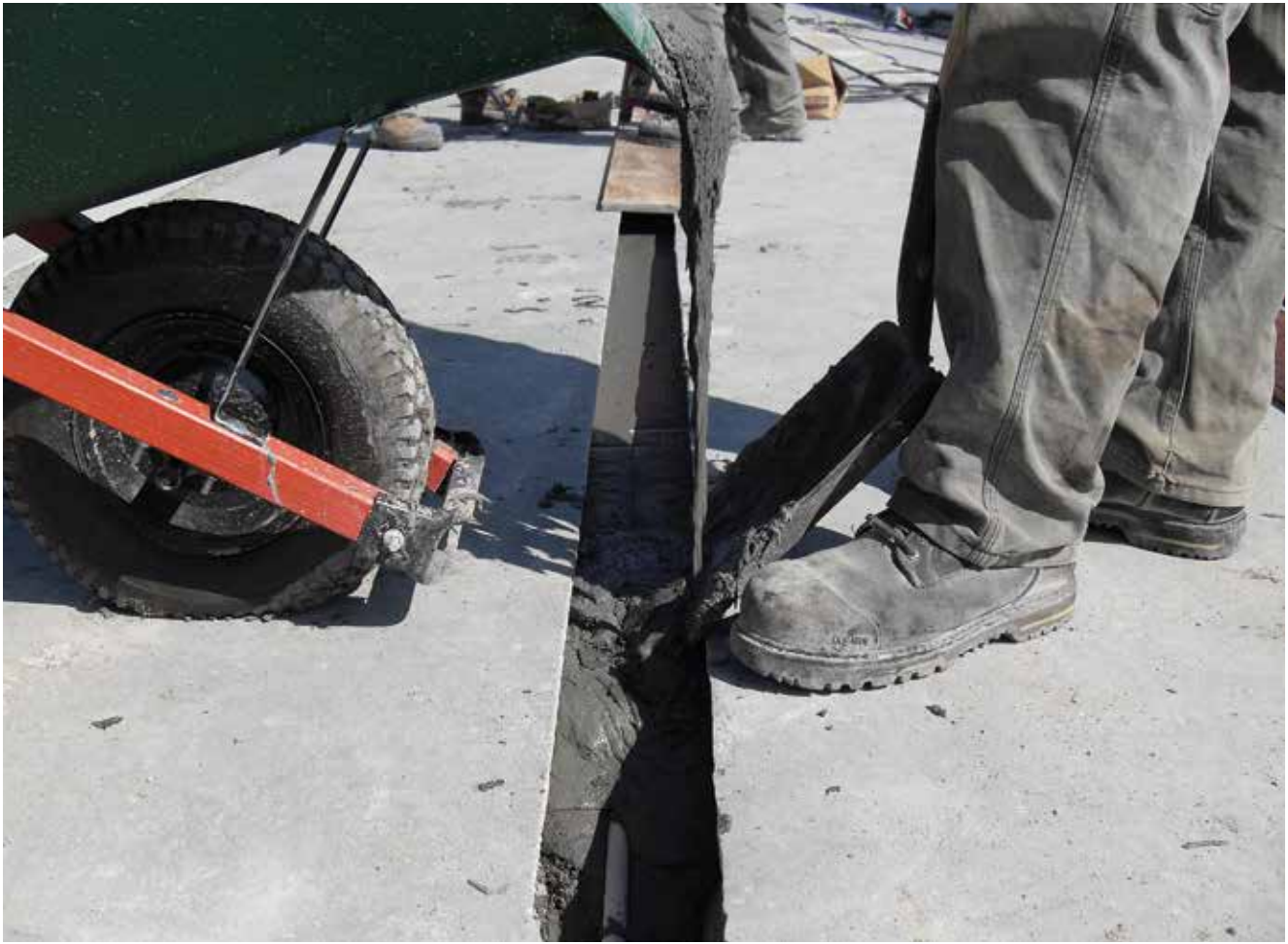
Figure 6. Placing the ultra-high-performance concrete material into a joint. Courtesy of Lafarge.
