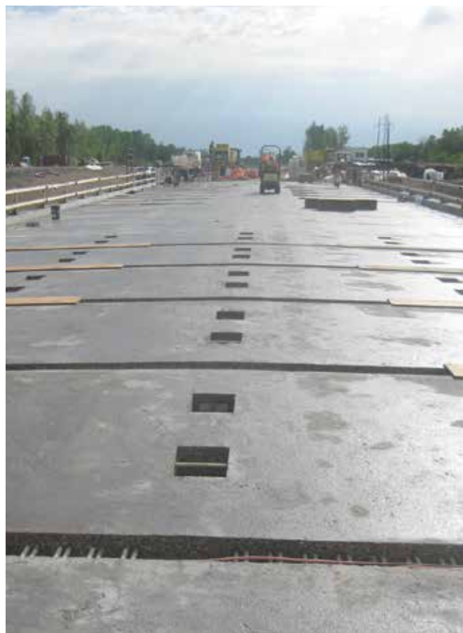
Figure 3. Full-width precast concrete deck panels ready for ultra-high-performance concrete joint fill. The concrete buggy in the upper portion of this photo is traveling along a previously completed section. Courtesy of Lafarge.
