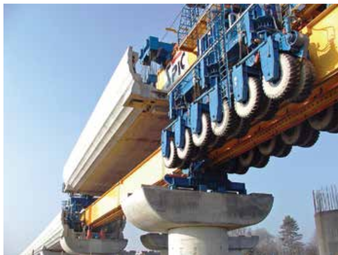
Figure 16. Portal carrier positioned for beam lowering.
