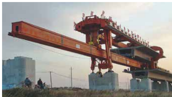
Figure 12. Short launcher with two-span underbridge for 32.7 m (107 ft), 9000 kN (2020 kip) dual-track box girders. Courtesy of BWM.
