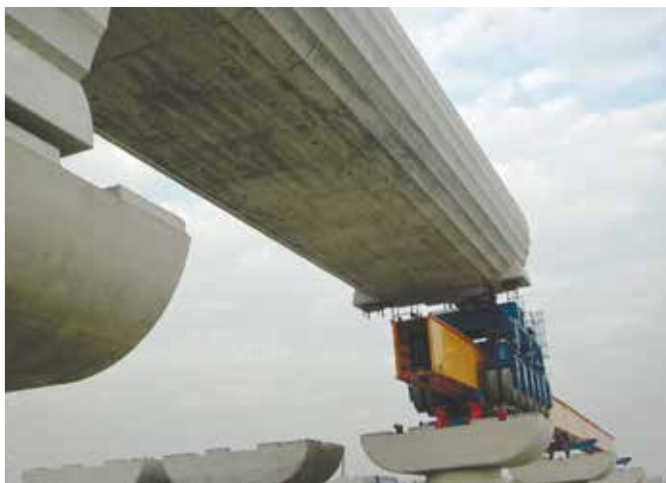
Figure 17. Repositioning the underbridge.
