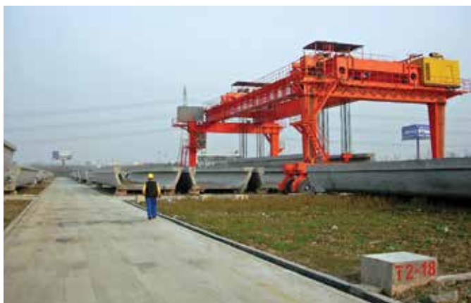
Figure 3. Large-scale storage of single-track U beams. Courtesy of Sysra.
