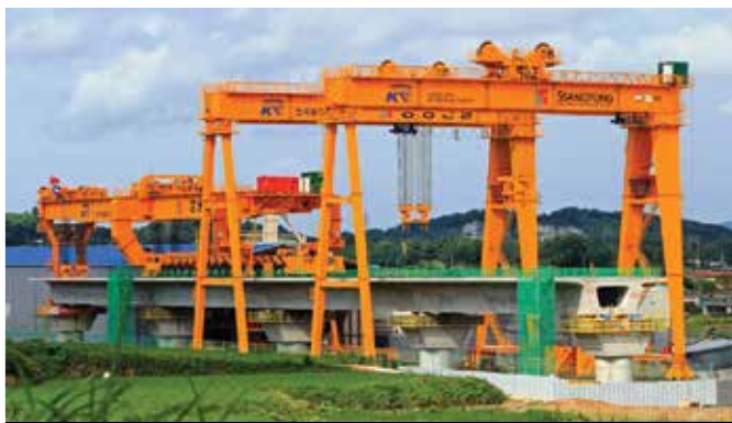
Figure 19. Four-beam assembly platform for elevated erection line. Photo courtesy of Struktur.
