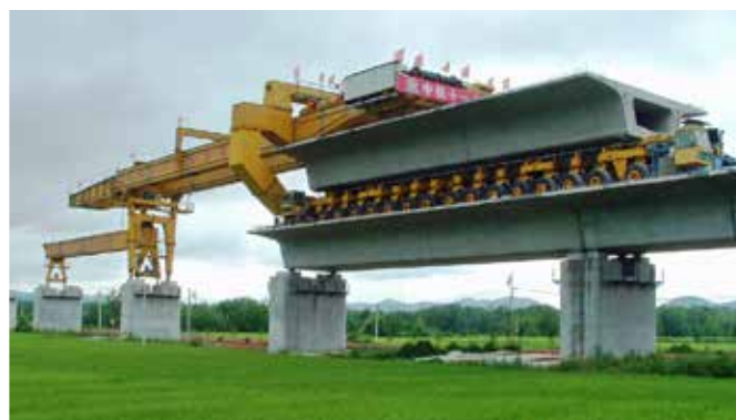
Figure 11. Telescopic beam launcher for 32.7 m (107 ft), 9000 kN (2020 kip) dual-track box girders. Courtesy of BWM.
