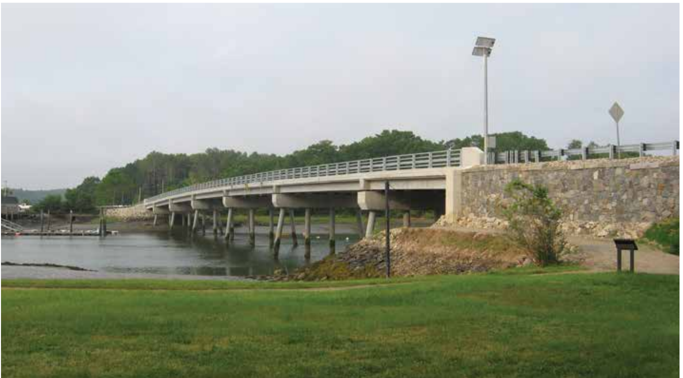
Figure 6. New Bridge in York, Maine.
