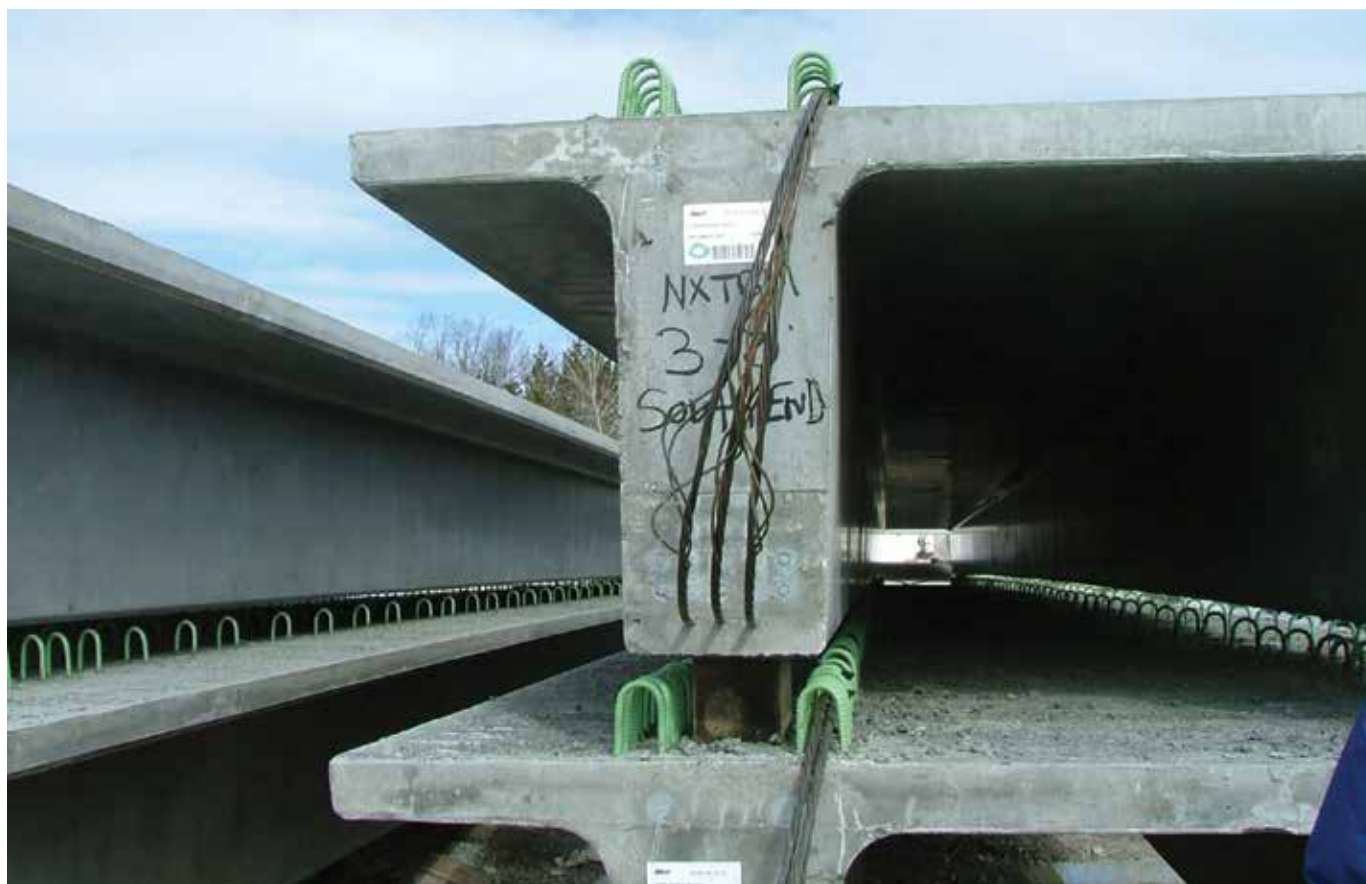
Figure 3. Stirrup placement.
