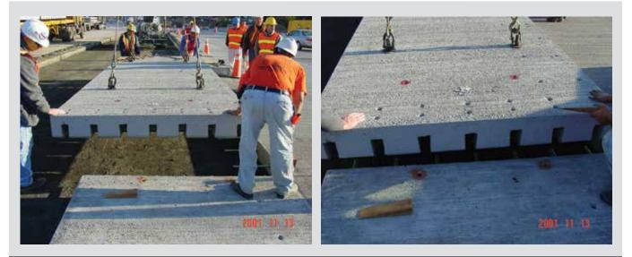
Figure 5. A scheme for providing load transfer in jointed precast concrete pavement.
