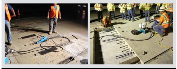
Figure 8. Views of the installation of two current versions of precast, prestressed concrete pavement systems.
