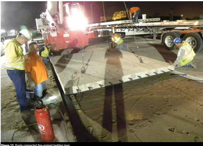
Figure 13. Poorly compacted fine-grained bedding layer.
