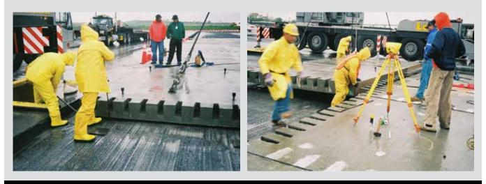
Figure 6. Alternative scheme for providing load transfer in jointed precast concrete pavement.
