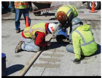
Figure 3. A variation for installing dowel bars using dowel bar retrofit.
