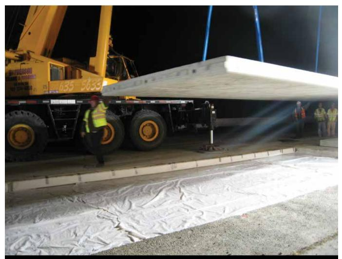
Figure 7. Installation of precast, posttensioned concrete pavement panels.
