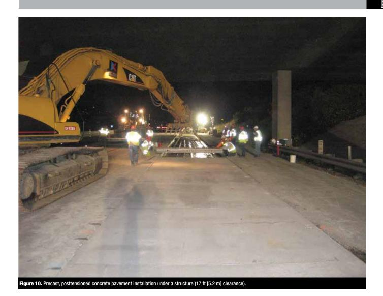
• Jointed precast, prestressed concrete pavement panels were installed in curved areas with radii ranging from 10,000 to 3200 ft (3000 to 980 m). Panels were fabricated in a casting bed that had flexible siderails and adjustable bulkheads.
