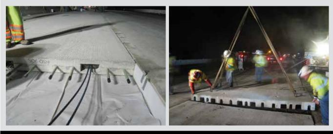
Figure 8. Final posttensioning and placement of temporary drop-in panel.
