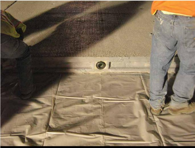
Figure 2. Keyway and 2 in. (50 mm) diameter posttensioning ducts between precast, posttensioned concrete pavement panels.
