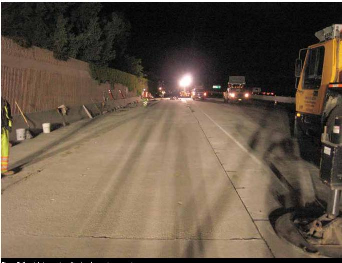
Figure 9. Completed precast, posttensioned concrete pavement.
