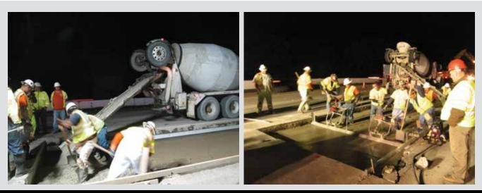
Figure 6. Placing and grading lean concrete base.
