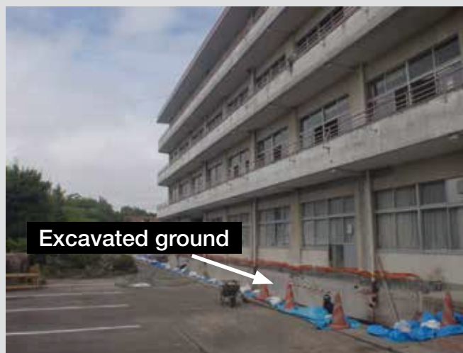
Excavation for newly installed foundation
