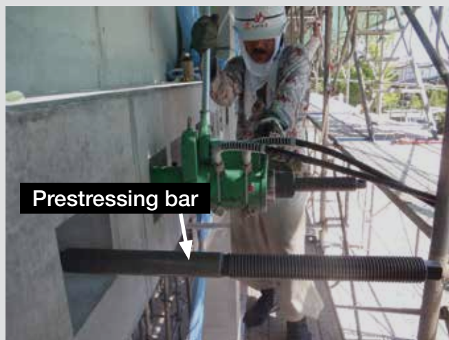
Connecting the parallel unit frame and the building with prestressing steel tendon
