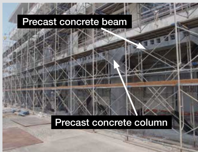
Assembly of precast concrete columns and beams
