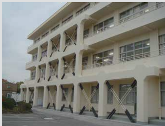
View after retrofit
