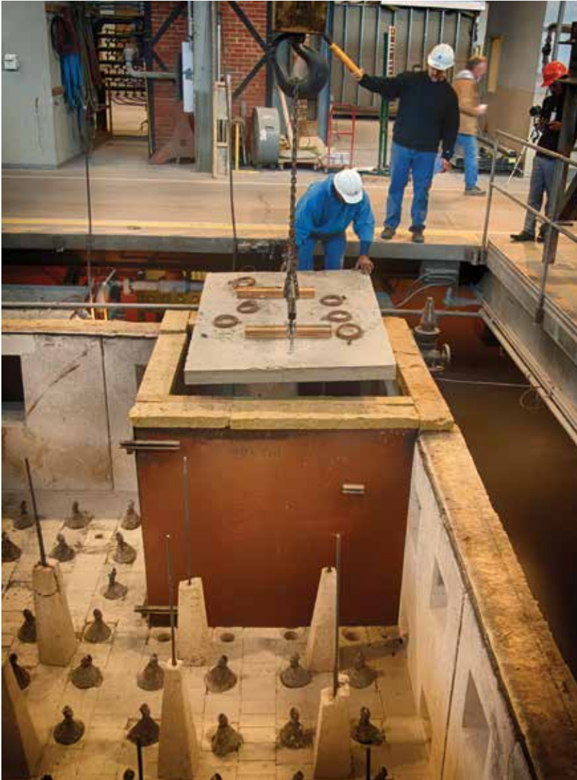
The test panel is lowered into place. Courtesy of Paul Grigonis.
