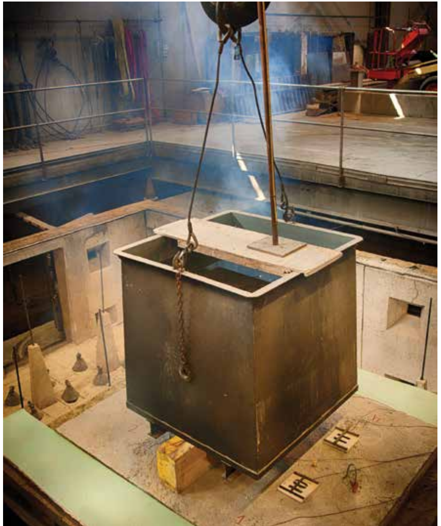
A water tank is lowered onto the slab as the preload. Courtesy of Paul Grigonis.
