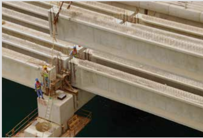
Precast concrete girders during erection
