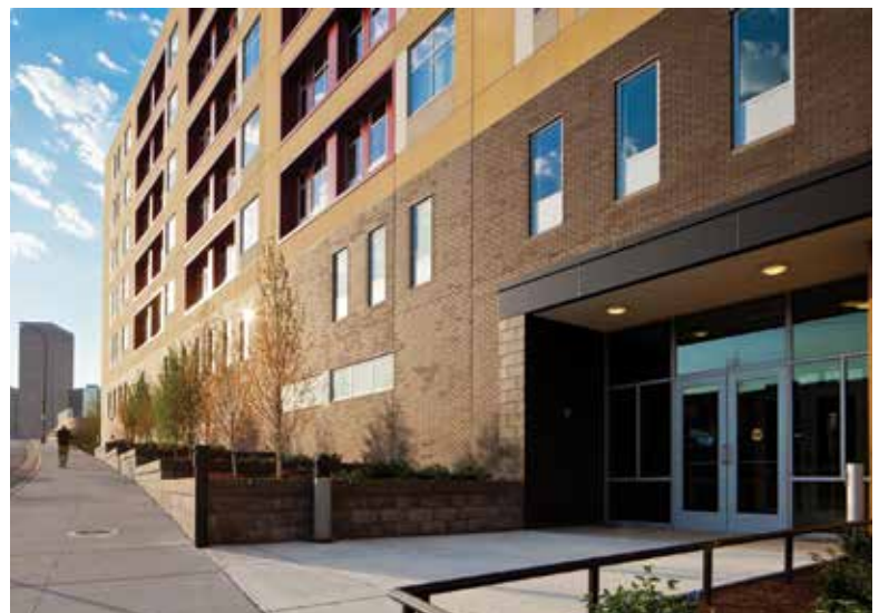
The Higher Ground homeless shelter is located on the edge of downtown Minneapolis, Minn. The first floor exterior features thin brick precast concrete cladding, except for a small area with concrete masonry units on two walls. The upper floors are clad in precast concrete sandwich wall panels with as many as three colors of concrete in one panel. Photograph by Brandon Stengel. Courtesy of Hanson Structural Precast.
