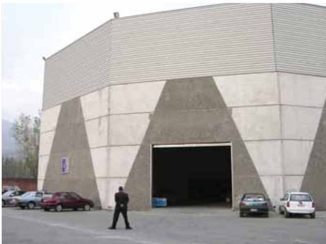
Figure 27. Annex of Preansa Convention Hall uses horizontal precast concrete panels.
