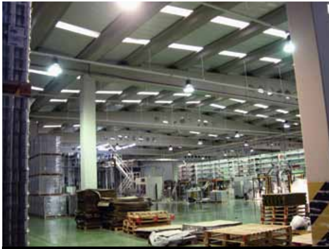
Figure 21. Interior view of the roof framing at a can factory.
