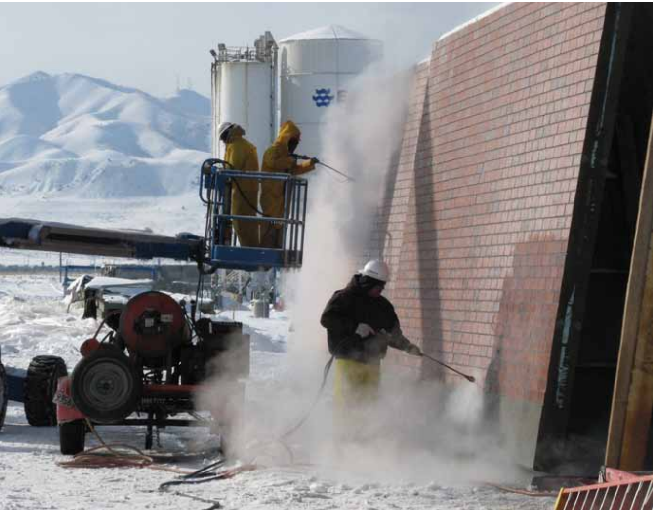
For the Fort Carson Brigade and Battalion Headquarters in Colorado Springs, Colo., EnCon had the precast concrete panels shipped early from its Salt Lake City, Utah, plant and finished at a local EnCon plant to avoid potential weather delays on the drive through the Rocky Mountains. Courtesy of Encon Utah.
