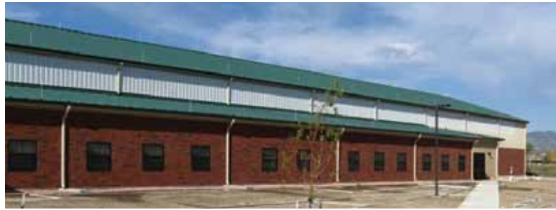
Reduced materials weight and waste contributed to the LEED gold certification of the Fort Carson Brigade and Battalion Headquarters in Colorado Springs, Colo. Courtesy of Chad Van Kampen/Encon Utah.
