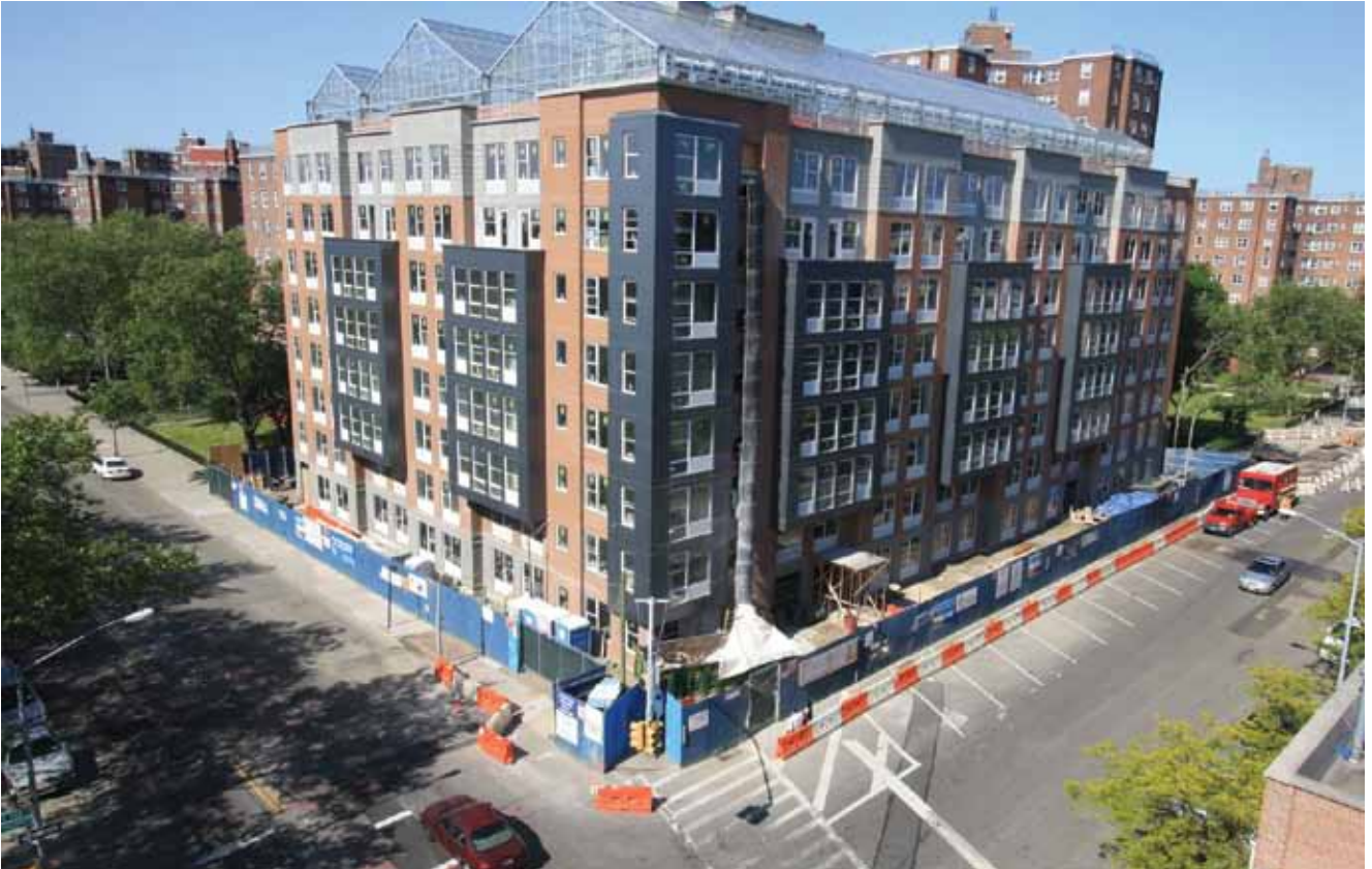
The Forest House apartment project in the Bronx, N.Y., uses precast concrete to gain many of its sustainable features. Oldcastle Building Systems helped work out the details of achieving a rooftop greenhouse, a filtered rainwater collection system, and better insulation for lower energy costs. Courtesy of Blue Sea Construction.
