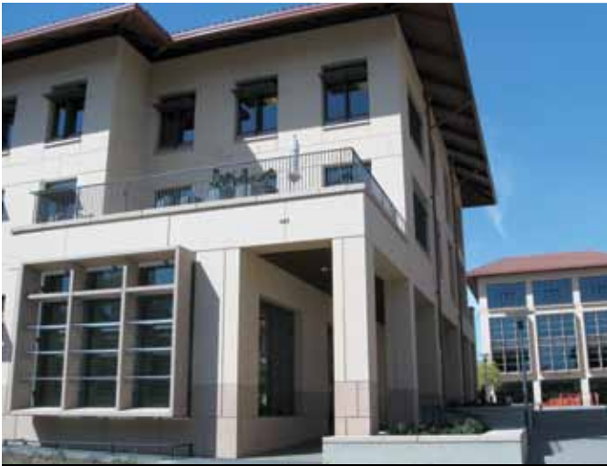
Figure 9. Glass-fiber-reinforced concrete in Stanford Graduate School of Business. Courtesy of Nippon Electric Glass America Inc.
