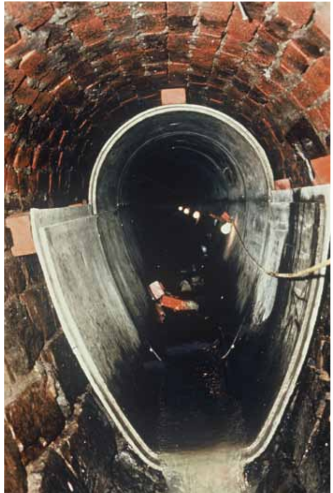
Figure 11. Glass-fiber-reinforced concrete sewer lining. Courtesy of Nippon Electric Glass America Inc.
