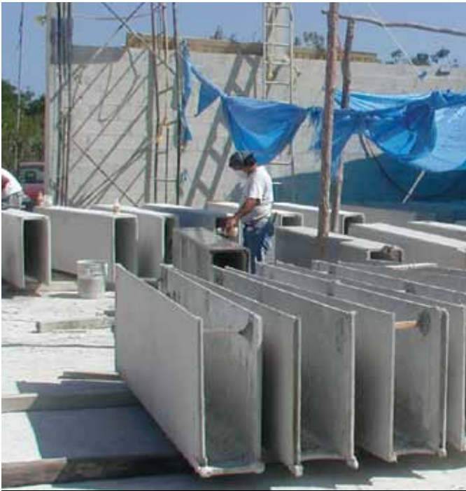
Figure 12. GFRC permanent formwork for beams in Puerto Rico. Courtesy of Nippon Electric Glass America Inc.
