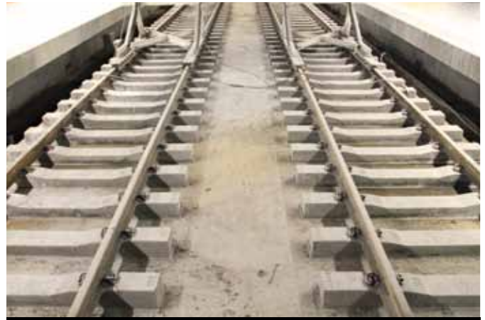
Figure 14. Precast concrete railroad track slabs for high-speed trains. Source: Brite-Euram (2002). Courtesy of Bekaert Corp. USA.
