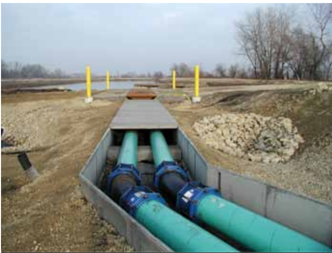
Figure 10. Glass-fiber-reinforced concrete pipeline trench application. Courtesy of Nippon Electric Glass America Inc.
