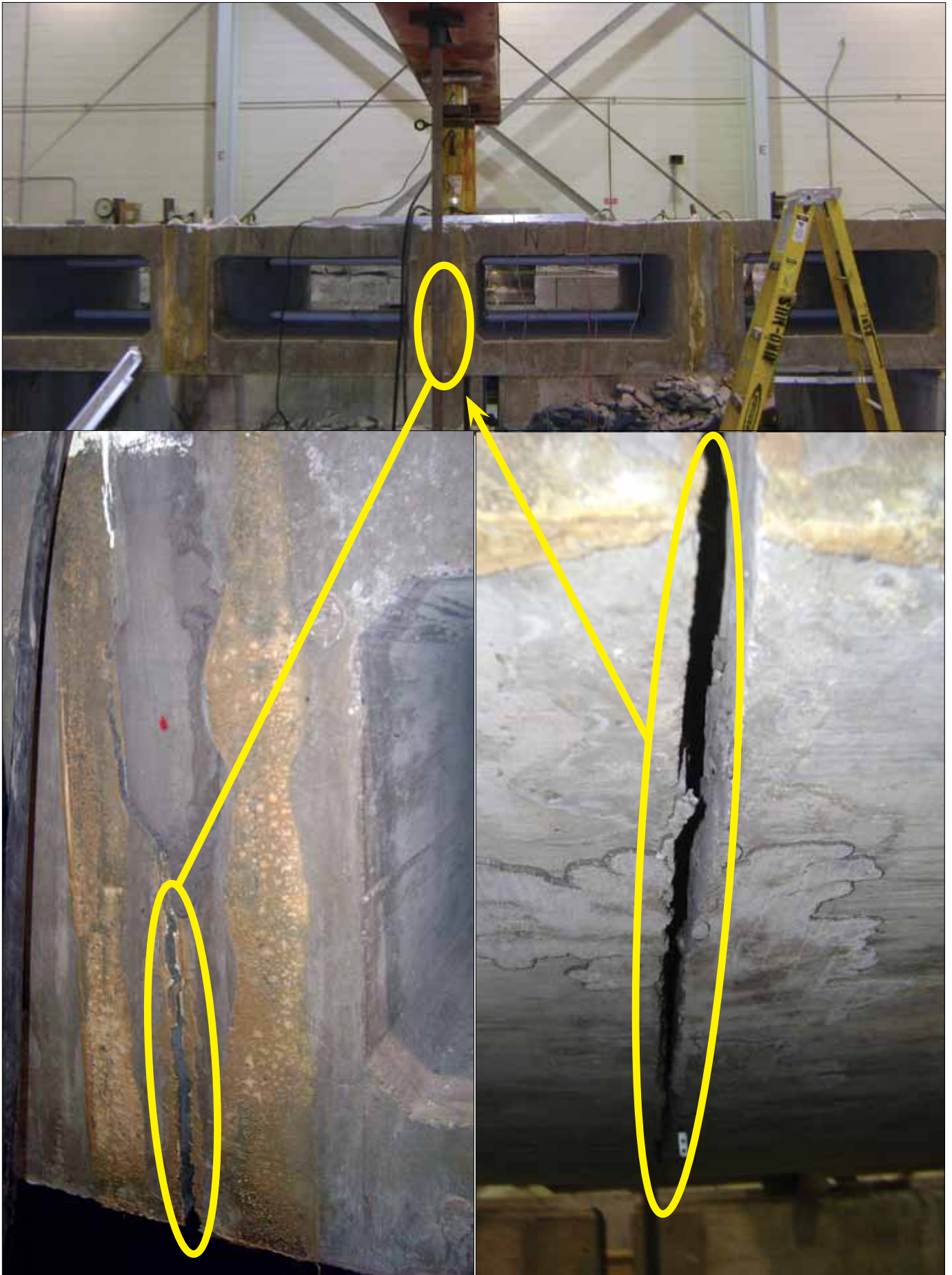
Figure 12. Side and underside cracking.
