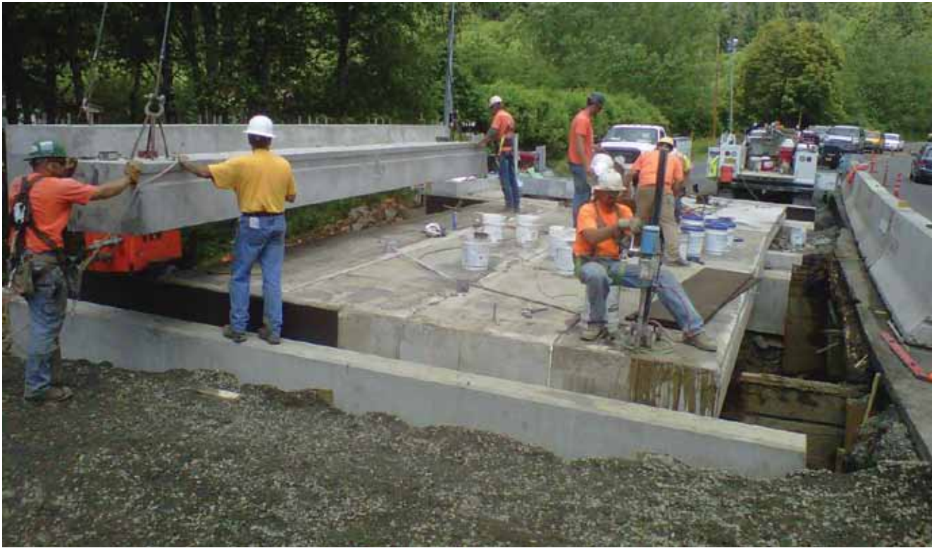
The old slab from an emergency detour bridge over Spencer Creek on Highway 101 in Oregon is being erected as part of the Volmer and Johnson Creek bridges project on US Route 26 between Portland, Ore., and the coast. The patches at the end of the slab indicate the locations where the strands were cut, recessed, and patched. Courtesy of Hamilton Construction Co.
