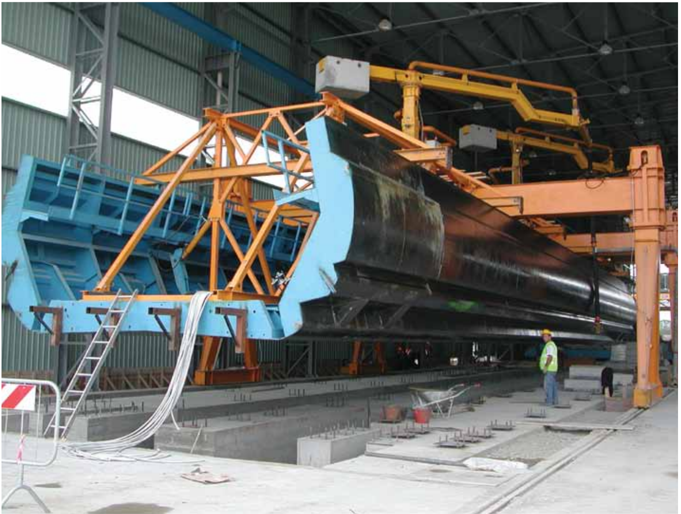
Figure 3. Movable interior form with concrete distribution arms.
