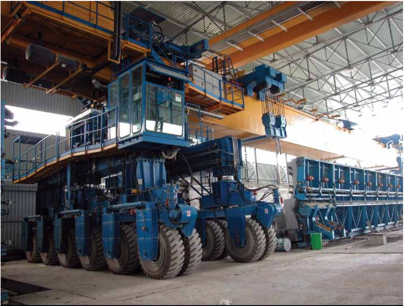
Figure 5. Span being lifted from the form.
