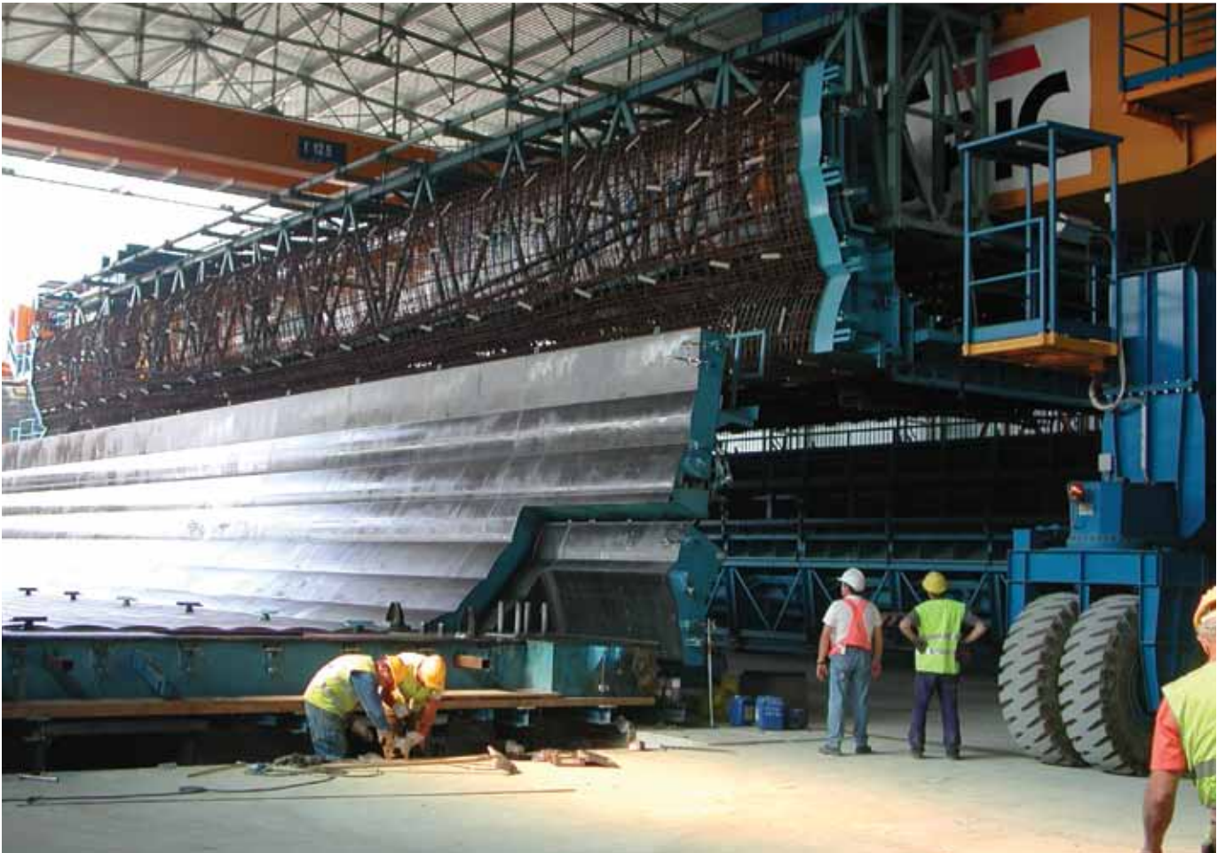
Figure 2. Cage delivery to the form.
