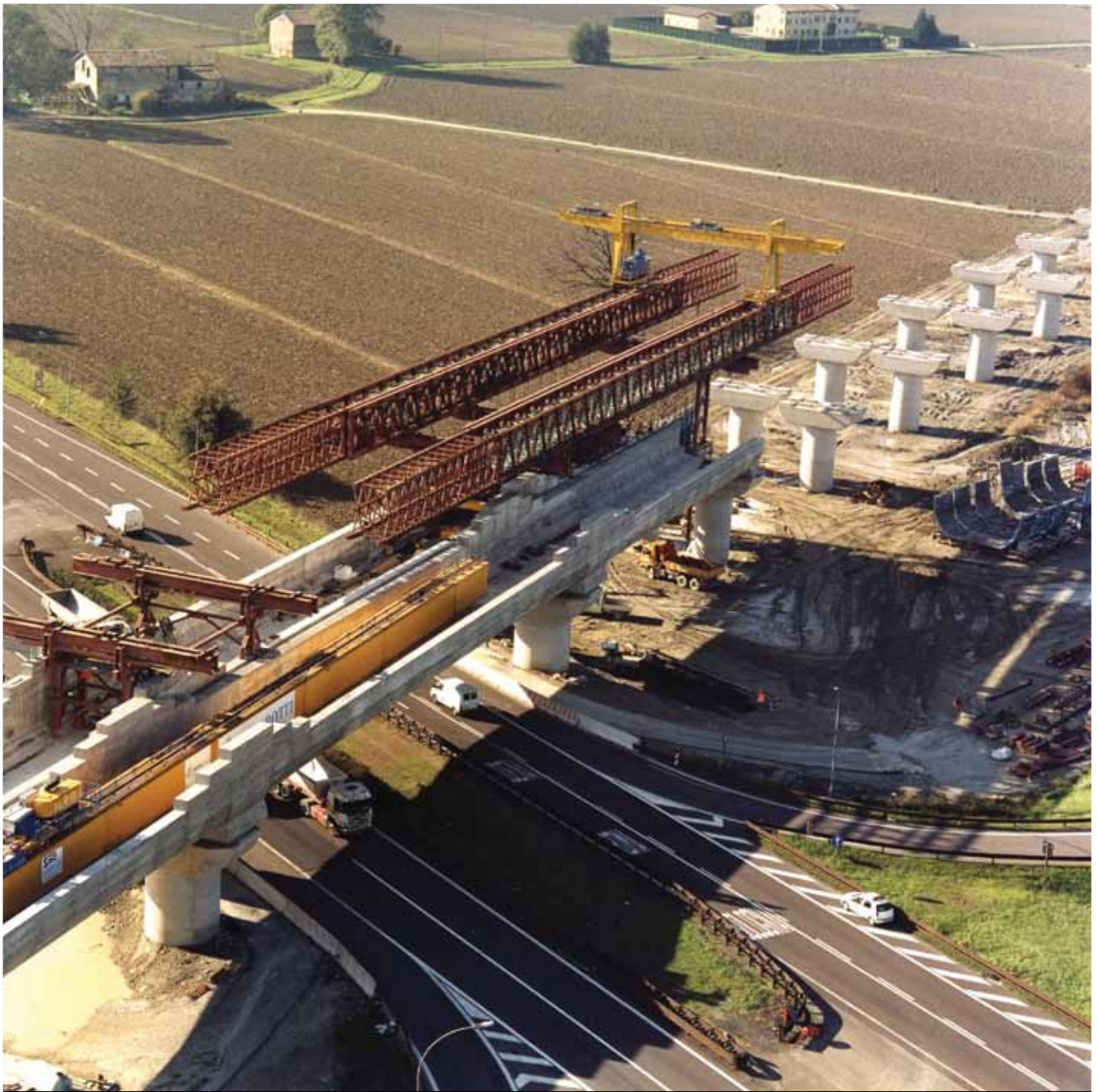
Figure 12. Main movable scaffolding system.
