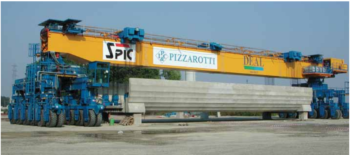
Figure 7. Span being lifted from the storage area.
