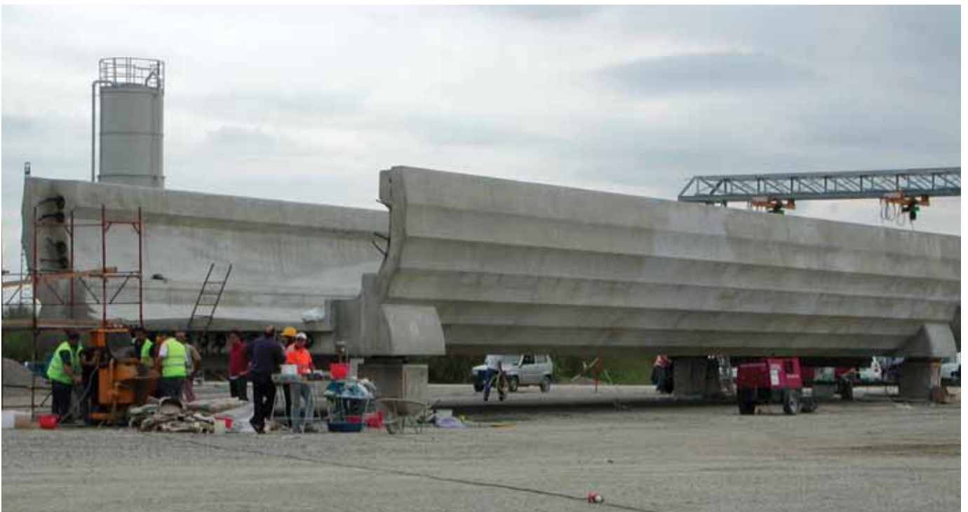
Figure 6. Span storage.
