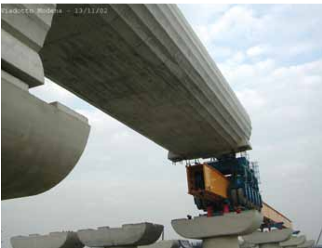
Figure 10. Forward launching of the underbridge.
