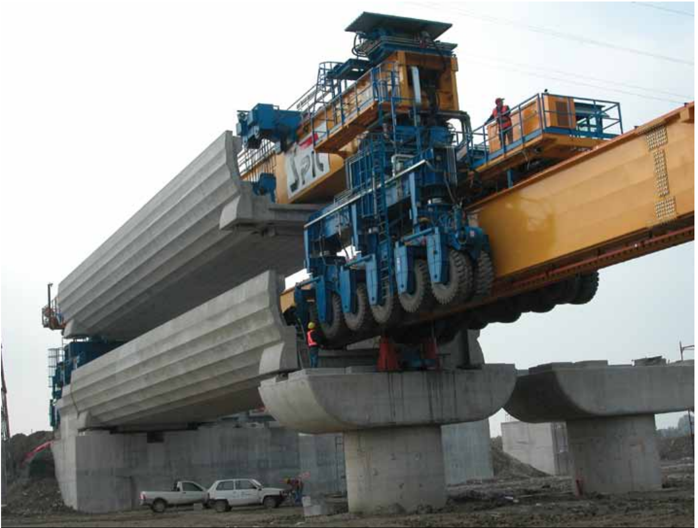
Figure 9. Front trolley advancing along the underbridge.
