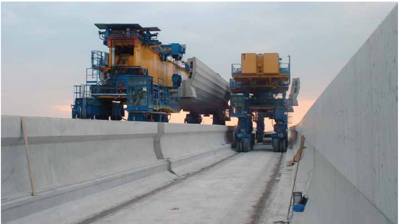
Figure 8. Span being transported.
