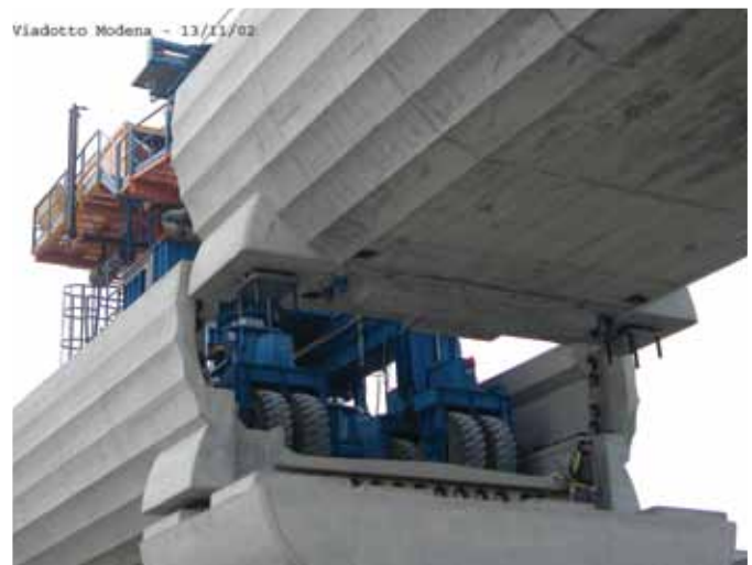
Figure 11. Final lowering of the span.
