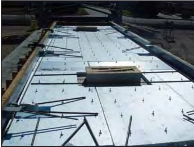
Figure 4.1.m. Blockout of foam around edge handling insert.
