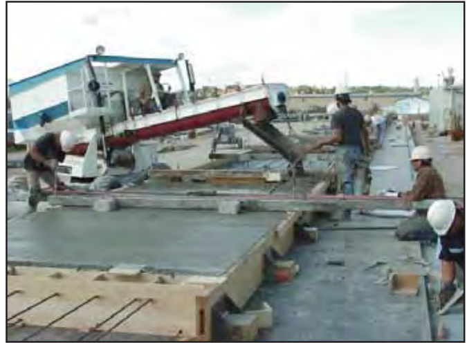
Figure 4.1.o. Placement of concrete backup over insulation. Use of pencil vibrator to consolidate backup mixture.
