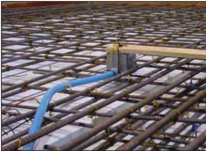
Figure 4.1.n. Electrical conduit and outlet box in place.
