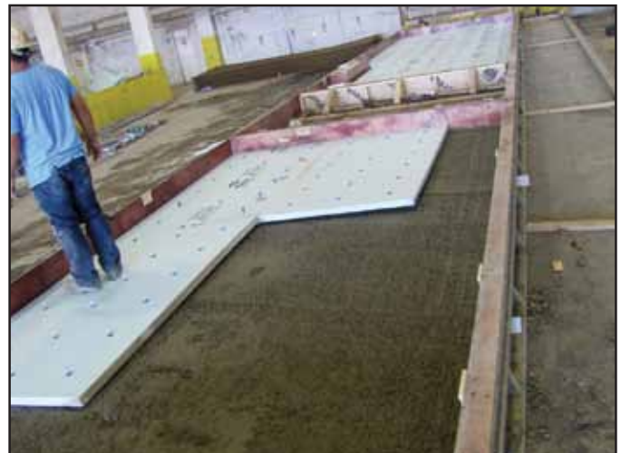
Figure 4.1.f. Insulation partially in place.
