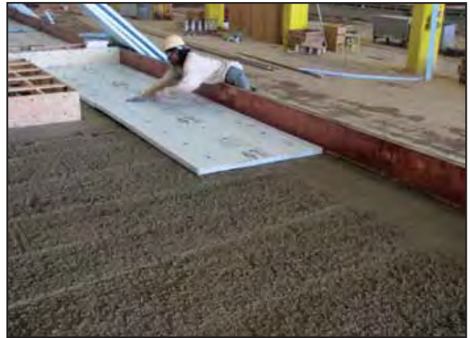
Figure 4.1.e. Placing 2-in.-thick (51 mm) insulation. Insulation can go outer edge to outer edge or can incorporate certain areas of panels that are uninsulated, depending on design criteria required.
