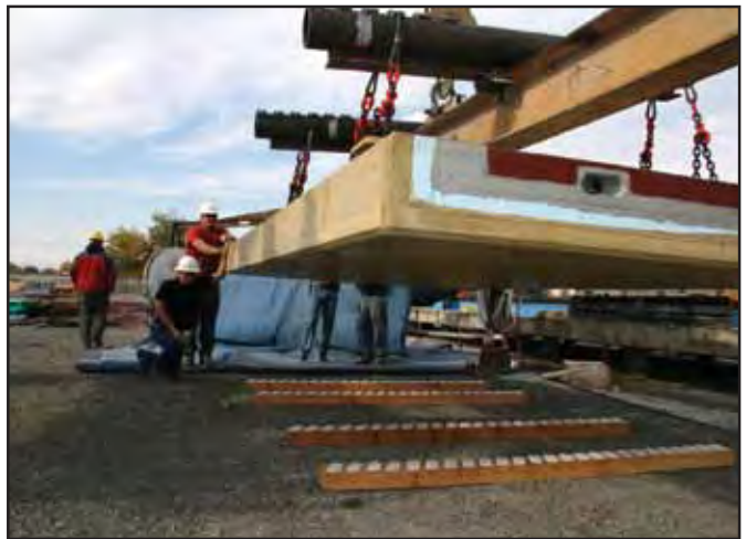
Figure 4.1.p. Stripping panel from form.
