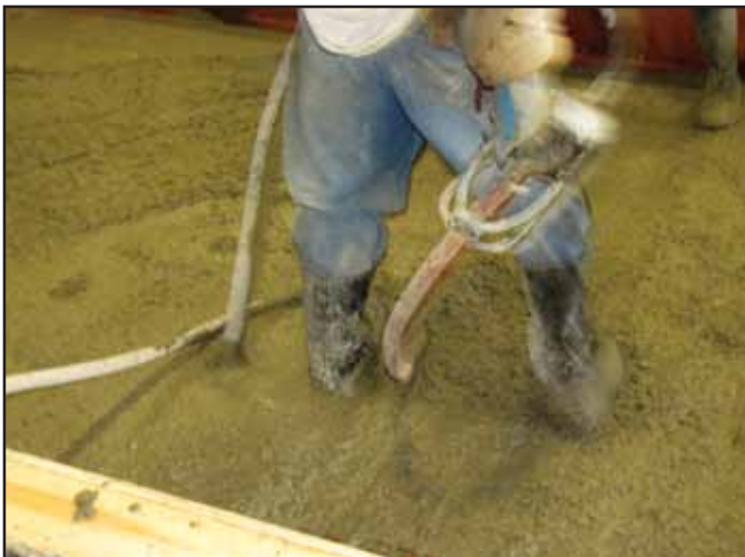
Figure 4.1.c. Vibrating face mixture using internal vibrator.
