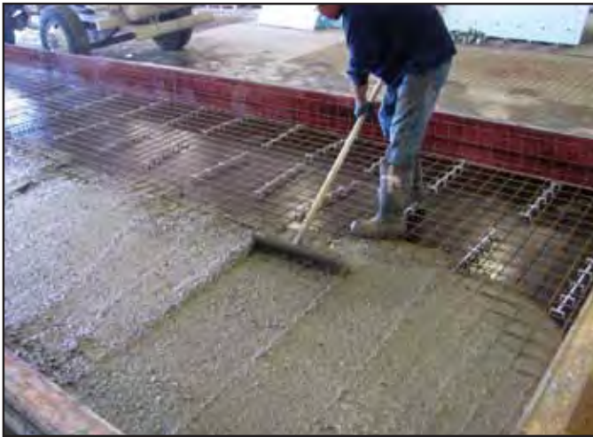
Figure 4.1.b. Concrete being placed as a part of face mixture, raking mixture to cover all surfaces of form. Once placed, concrete will be vibrated with both external and internal units; placement depth is 3 in. (76 mm) for face mixture.
