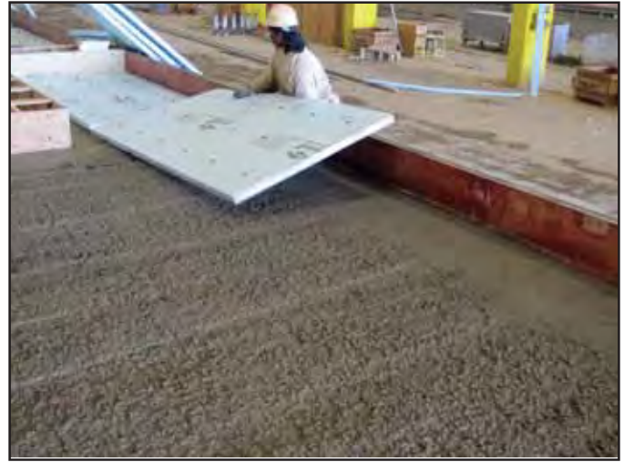
Figure 4.1.d. Placing 2-in.-thick (51 mm) insulation. Insulation is predrilled at 16 in. (406 mm) on center to accept pin-style connectors.
