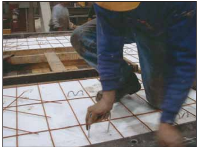
Figure 4.1.j. Stainless steel pin connectors for connecting wythes.
