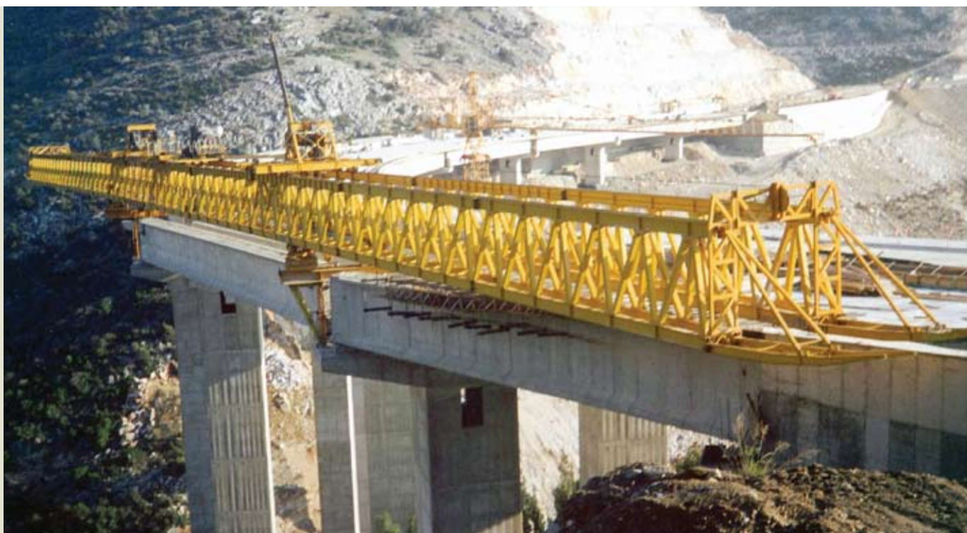
Figure 2. The edge girder is being placed. Photograph courtesy of Comtec.
