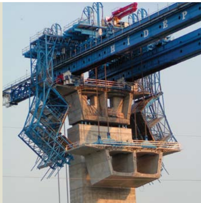
Figure 12. Strand-jack lifting of macrosegments is used for balanced-cantilever construction. Photograph courtesy of Thyssenkrupp.
