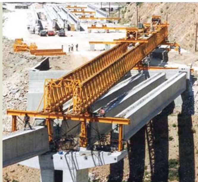
Figure 1. This light gantry is used for precast concrete girders. Photograph courtesy of Comtec.
