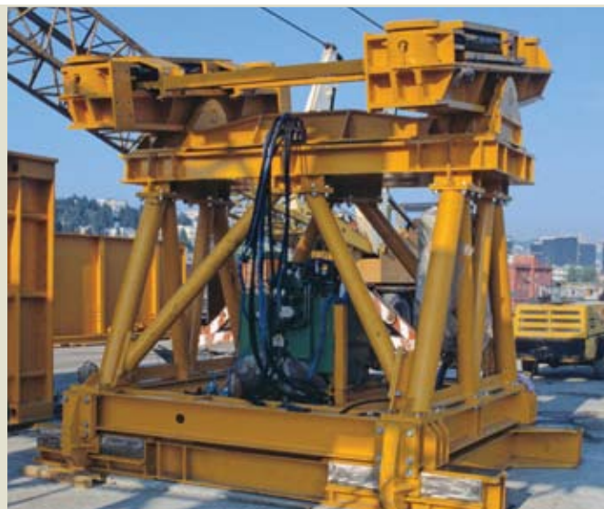
Figure 6. A friction launcher is assembled onto a support tower.
