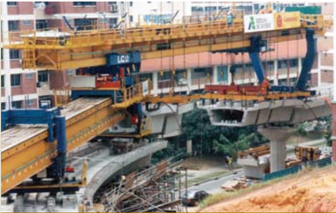
Figure 8. This is the pivoted single-upper-beam gantry for curved precast concrete segmental bridges. Photograph courtesy of Deal.
