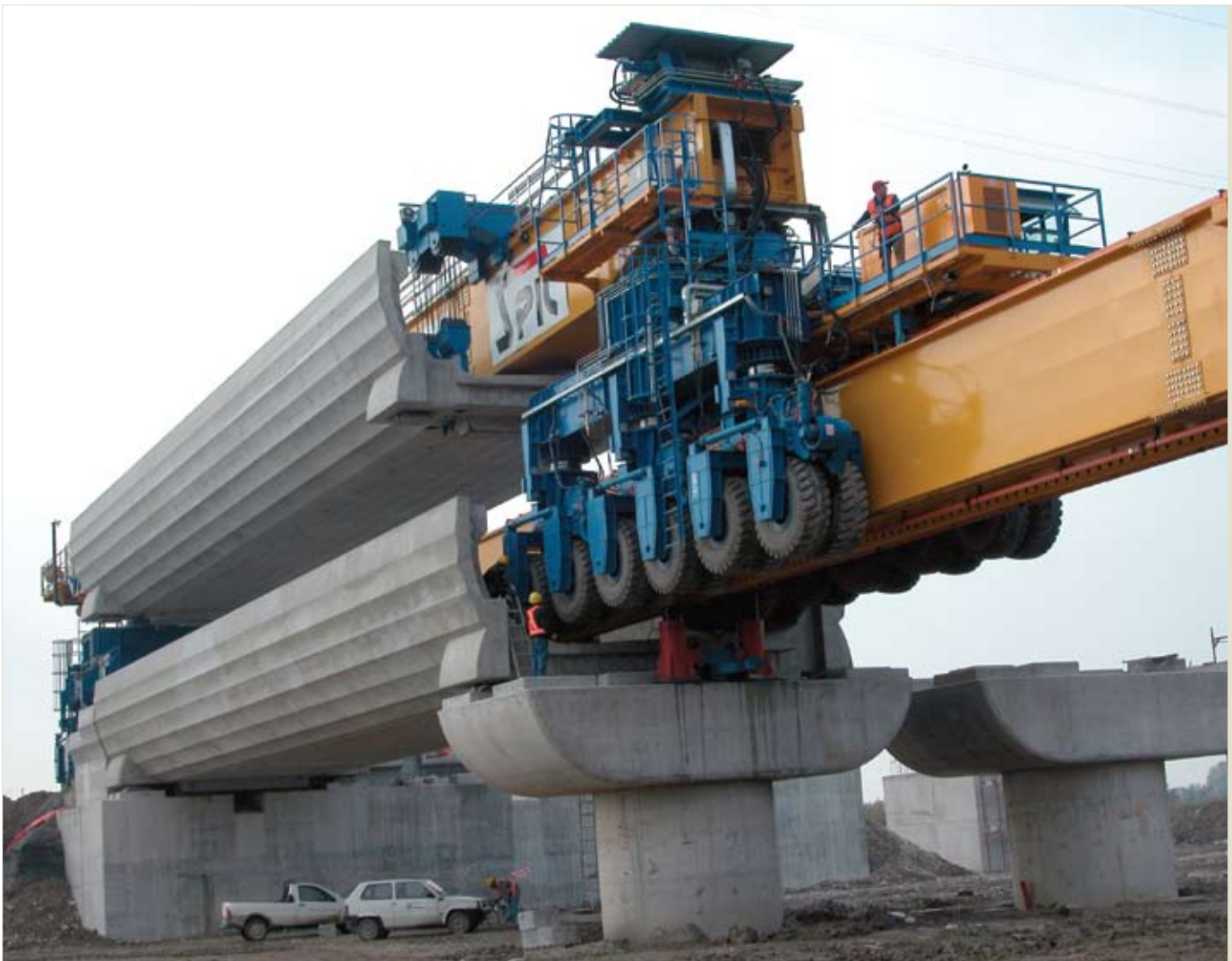
Figure 14. This wheeled span carrier has a self-launching support beam for high-speed railway projects.
