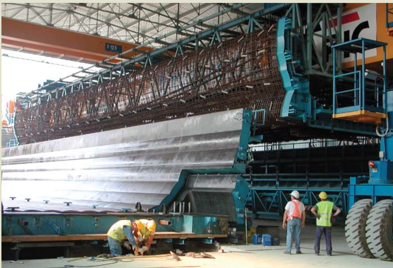
Figure 13. The prefabricated cage for the entire span is being inserted into the casting cell.
