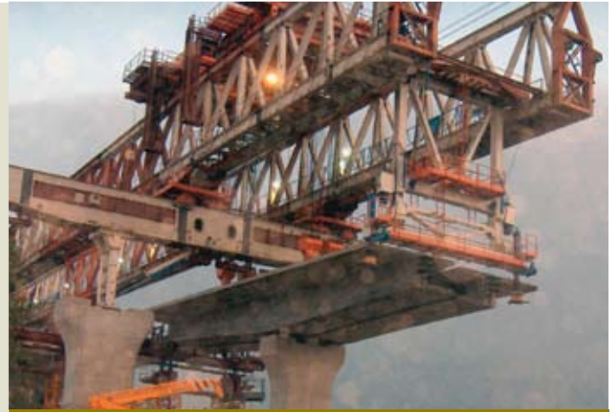
Figure 9. This heavy twin-upper-truss unit is for precast concrete macrosegmental erection.
