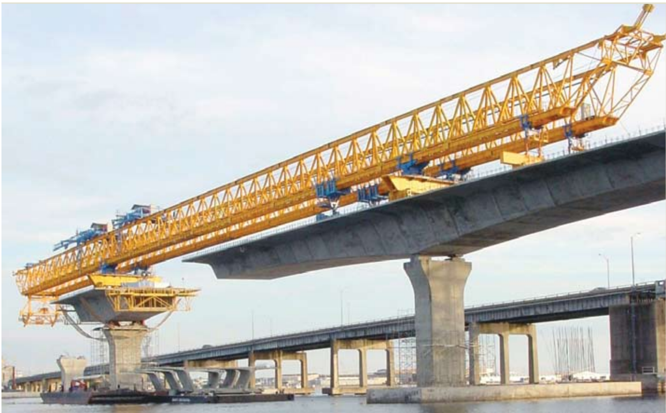
Figure 10. This long twin-upper-beam gantry is used for balanced-cantilever erection. Photograph courtesy of HNTB archive.
