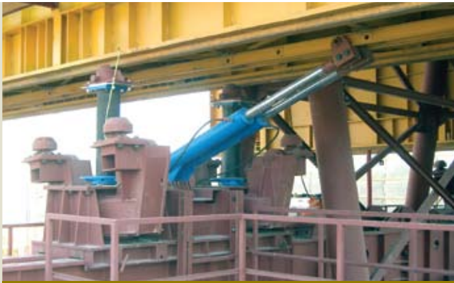
Figure 4. The launch cylinders of a twin-lower-beam gantry are shown in the raised configuration for segment assembly.
