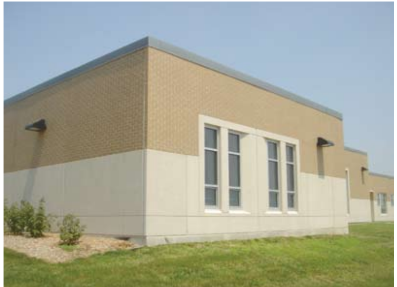
IPC Inc. provided precast concrete for the renovation of the Blue Valley Academy in Stanley, Kans. Courtesy of IPC Inc.
