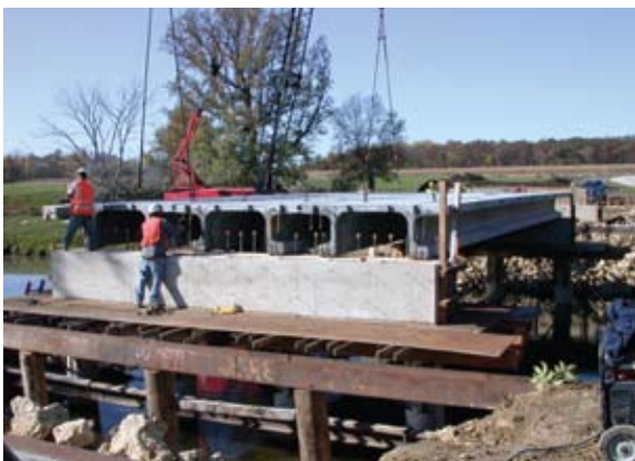
The Jakway Park Bridge in Buchanan County, Iowa, uses pi-girders made with ultra-high-performance concrete to make the bridge more durable. Courtesy of Iowa Department of Transportation.
