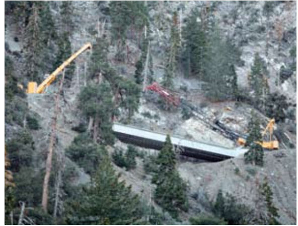
The Angeles Crest Bridge No. 1 on state route 2 in Wrightwood, Calif., pitted designers against location and weather challenges. Courtesy of Pomeroy.
