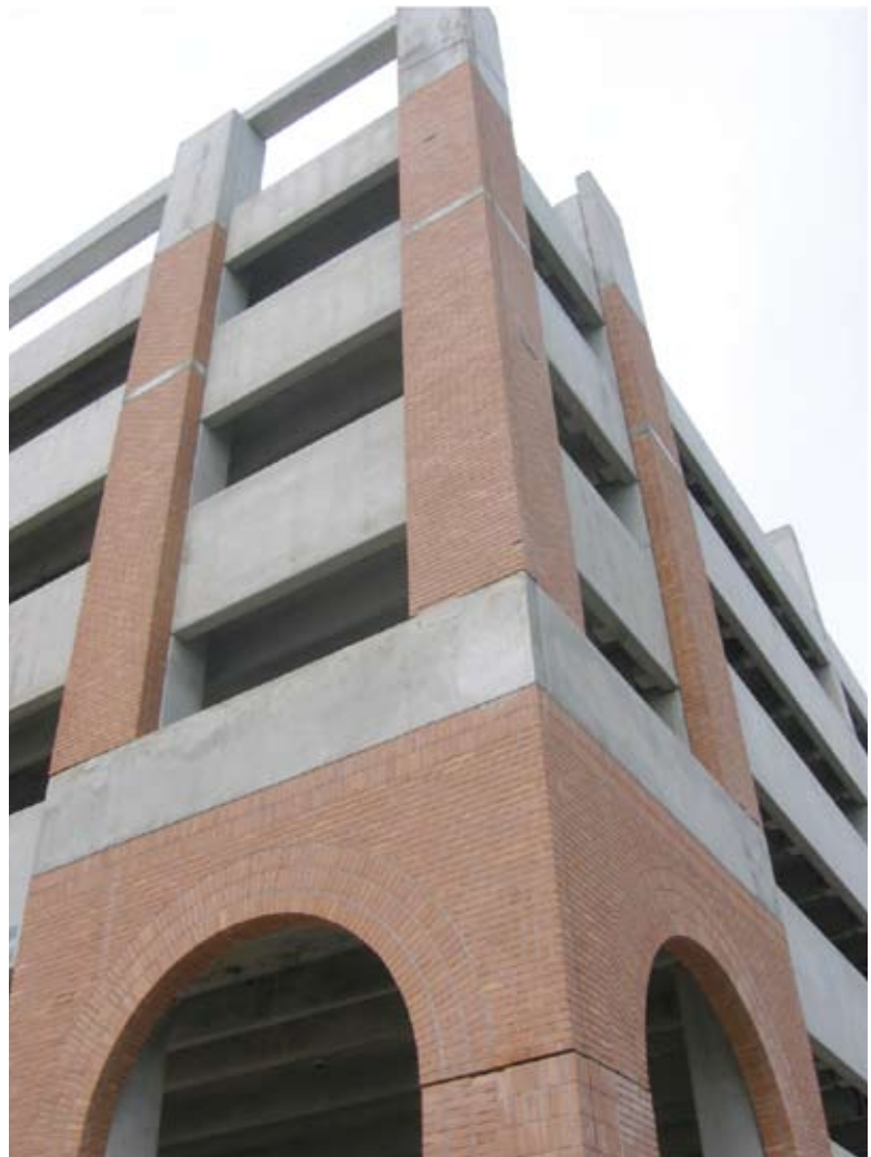
The Destin Commons West parking structure received the Florida Parking Association's 2008 Award of Excellence. Courtesy of Walker Parking Consultants Inc.
