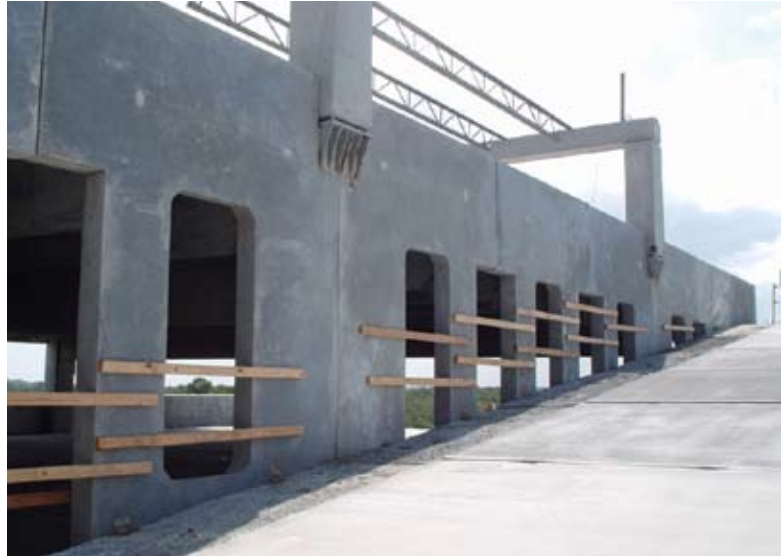
Parking deck wall panels support the precast concrete office frames of the Destin Commons West parking structure in Destin, Fla. Courtesy of Walker Parking Consultants Inc.
