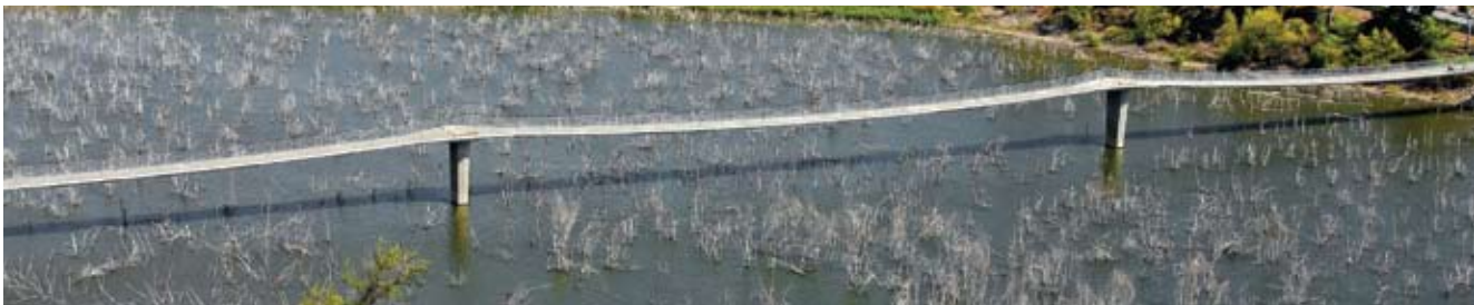
As the longest stress-ribbon bridge in the world, the precast concrete David Kreitzer Lake Hodges Bicycle Pedestrian Bridge in San Diego, Calif., spans an environmentally protected lake. Courtesy of Mark Defeo.
