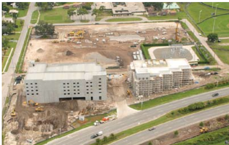
The fast-tracked Tripointe Plaza Garage in Tampa, Fla., is being erected in a small, tight location. Photo courtesy of Coreslab Structures (TAMPA) Inc.
