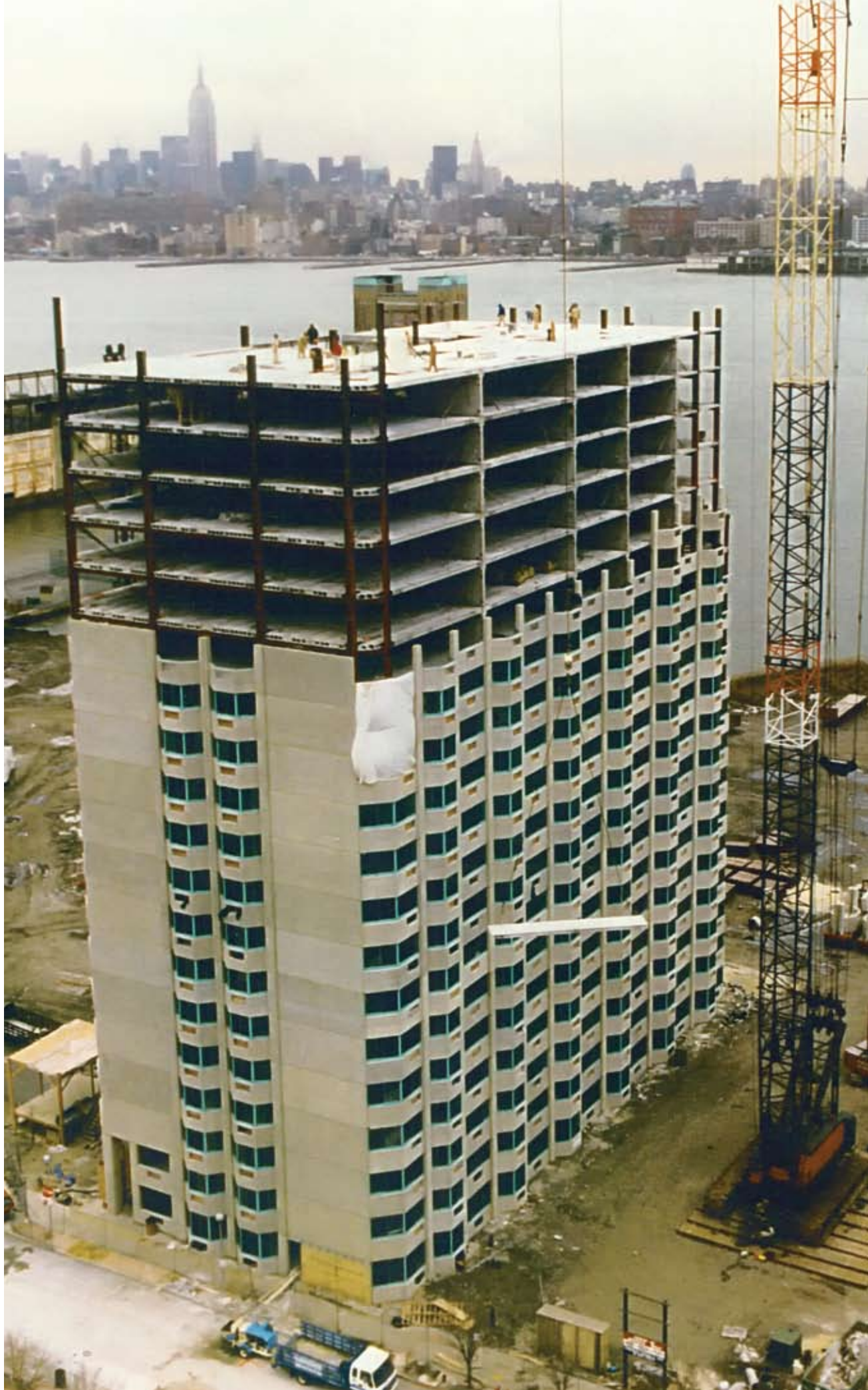
Erection at the 20th story of the Tower of America West in Jersey City, N.J., is performed with a larger crawler crane. Photo courtesy of Tower of America Urban Renewal Co.
