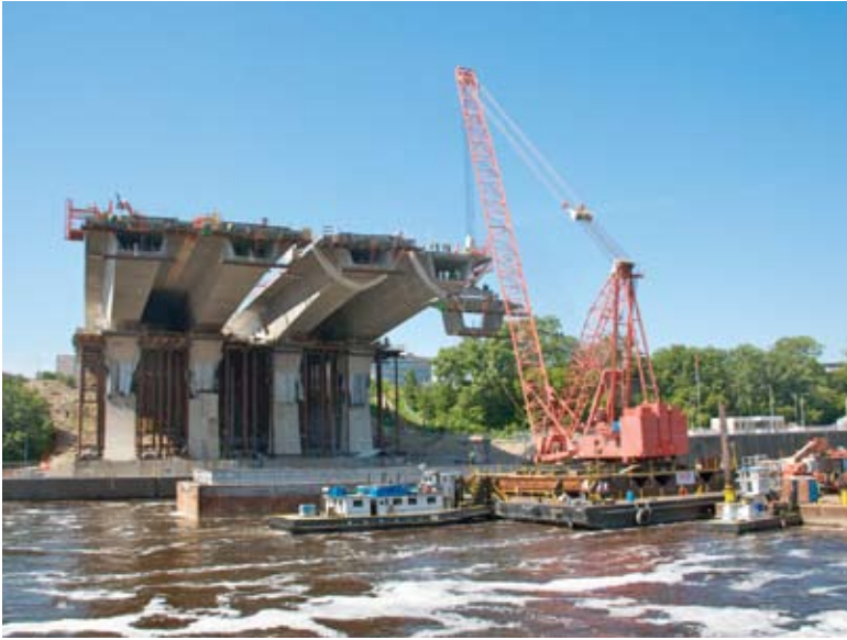
Erection began on the 504 ft (154 m) main span of the St. Anthony Falls Bridge over the Mississippi River in Minneapolis, Minn., on May 25, 2008, and was completed on July 10, just 47 days later. Typically, four segments were set each day. Courtesy of FIGG, Tim Davis photographer.
