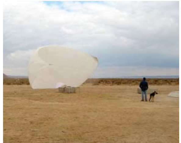
California State Polytechnic University, Pomona, students use a kite to move precast concrete blocks while erecting a pyramid. Courtesy of Doug Mooradian.
