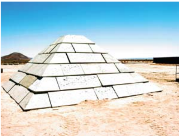
The top of a pyramid assembled by California State Polytechnic University, Pomona, students using kites to lift the stones is all that is left to complete the project. Courtesy of Doug Mooradian.
