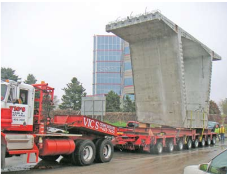
The four parallel box girders in the 504 ft (154 m) main span of the St. Anthony Falls Bridge required 120 precast concrete segments. Upon completion of casting, the segments, weighing up to 200 tons (180 tonnes), were moved to a site next to the river, then loaded onto barges for erection in the main span. Courtesy of FIGG, Tim Davis photographer.
