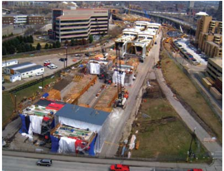
Eight long-line casting beds were established on the unused Interstate 35W roadbed, just south of the St. Anthony Falls Bridge site in Minneapolis, Minn. Rolling, heated enclosures facilitated casting segments through Minnesota winter weather. Courtesy of FIGG, Tim Davis photographer.
