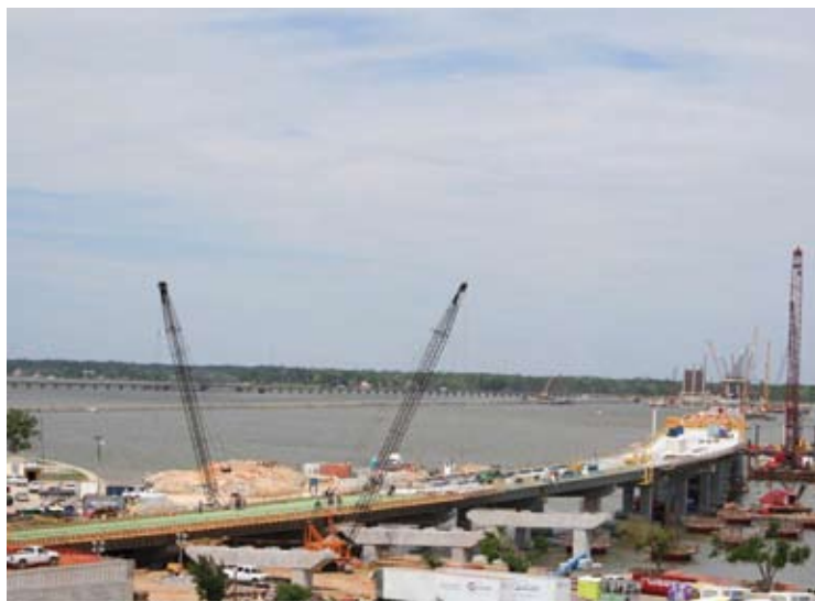
The westbound lanes of the north section of the Biloxi Bay Bridge in Mississippi were completed first and opened 12 days ahead of schedule. At peak construction, 18 floating cranes were on site. Courtesy of Mississippi Department of Transportation.
