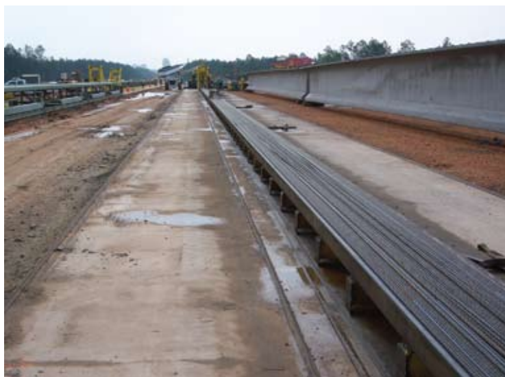
The prestressed rolling system used in the Biloxi Bay Bridge in Mississippi allows forms to be moved and reset in just 30 minutes. Courtesy of Mississippi Department of Transportation.
