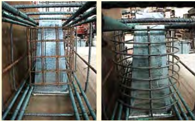
Welded-wire reinforcement
