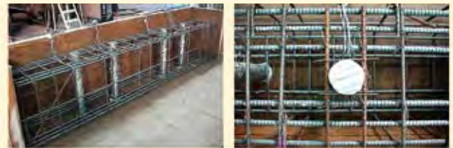
Ducts in reinforcement cage
