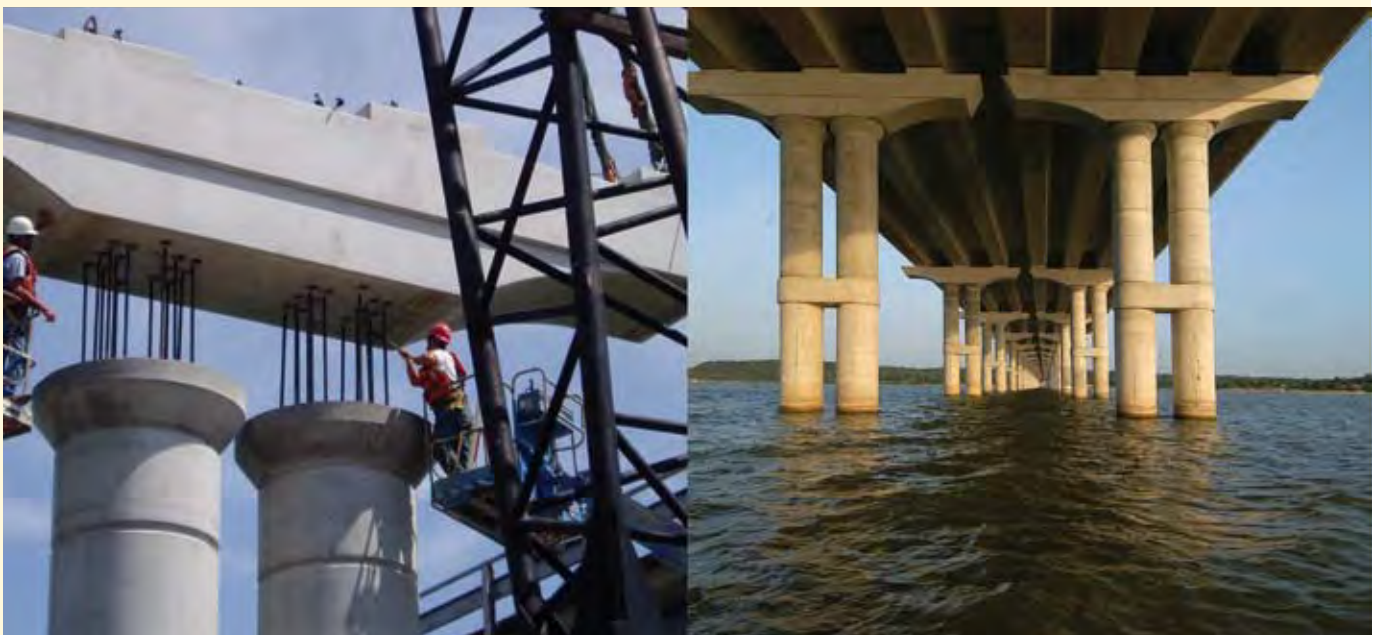
Lowering of precast concrete bent cap
