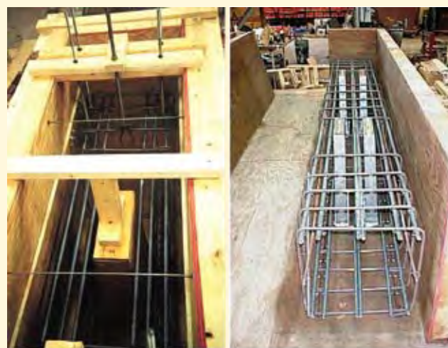
Single-line grout pocket
