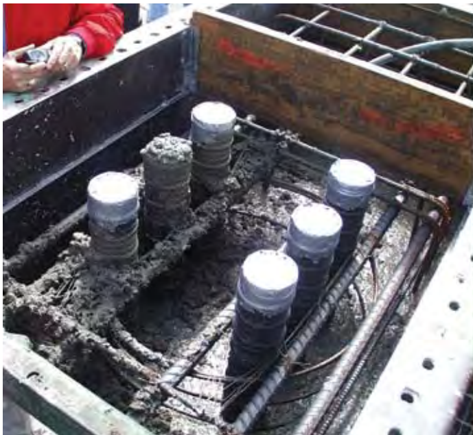
Precasting of concrete bent cap using grouted-duct connection
