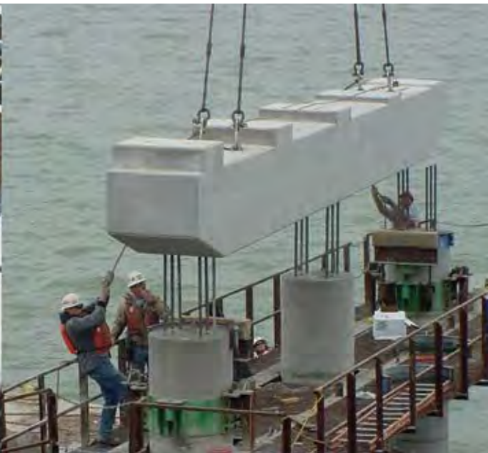
Lowering of precast concrete bent cap onto friction collars
