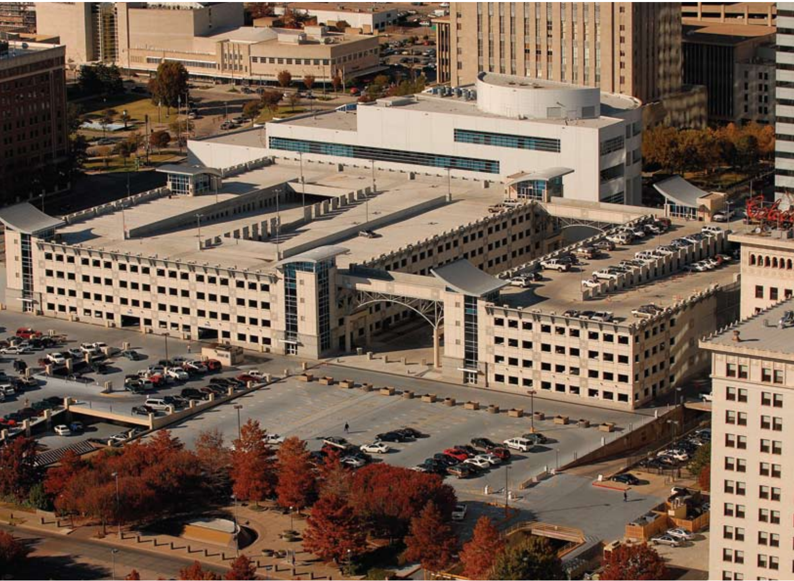
This aerial photo shows the completed City Center Parking Facility in Oklahoma City, Okla. Courtesy of the City of Oklahoma City.
