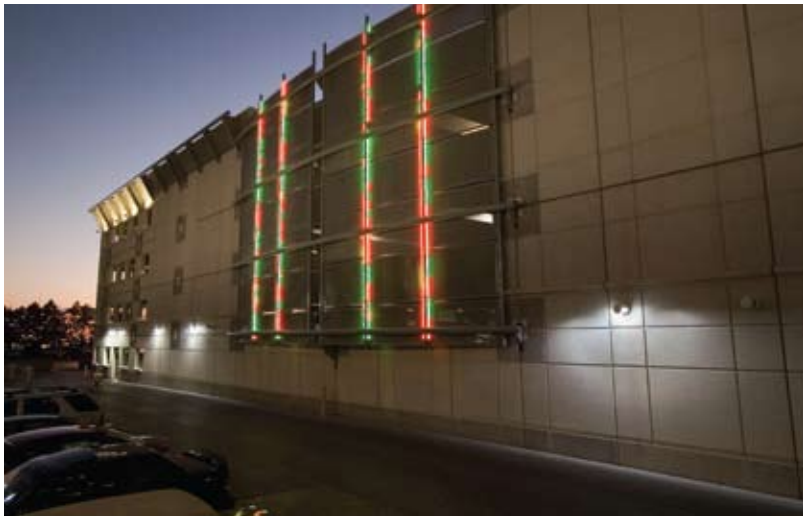
Lower right As part of the aerodynamic automobile design of the City Center Parking Facility in Oklahoma City, the perforated metal-screen panel on the east facade is designed to mimic the front-end grill of a classic Mercedes sedan and serves to conceal sloped ramping. Courtesy of Quinton Myers, copyright: ADG.
