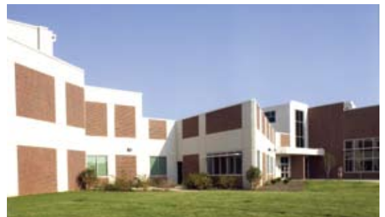
From top This outside view of Riverside High School in Greer, S.C., shows the building's fenestration. Courtesy of BRPH Cos. Inc. of Marietta, Ga.
