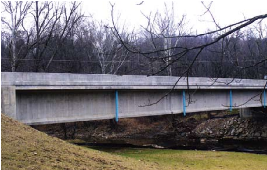
Side view of new Jeff Danzer Bridge over the Little Scioto River.
