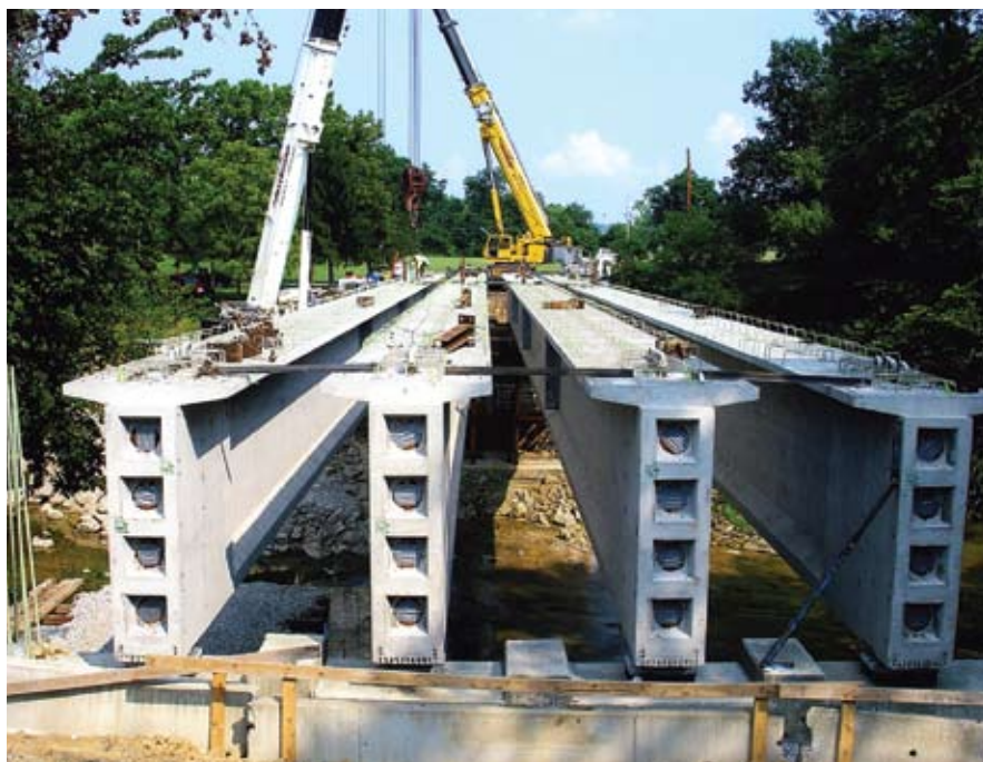
Newly installed, precast concrete bulb-tee girders.
