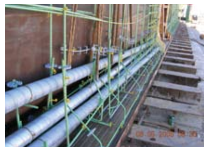
Swept ducts in girders prior to concrete placement.
