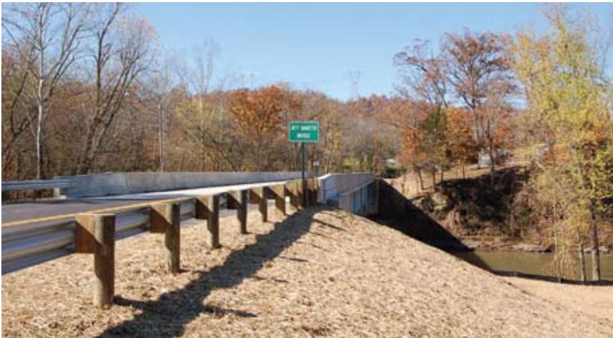
Top view of new Jeff Danzer Bridge over the Little Scioto River.
