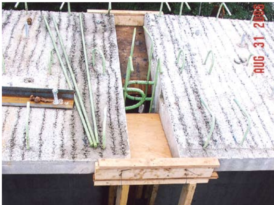
Adjoining precast concrete bulb-tee girder sections showing 1 ft (0.3 m) closure joint.
