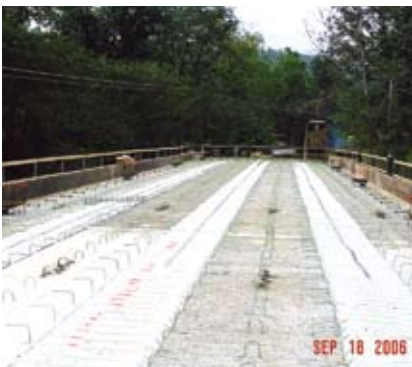
Bridge surface ready for 8½-in.-thick (216 mm) deck slab.
