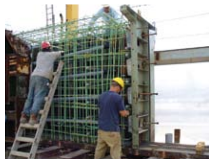
End girder detail prior to placing concrete in the girder.
