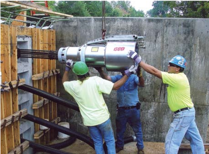
Post-tensioning the precast concrete bulb-tee girder at bridge end.
