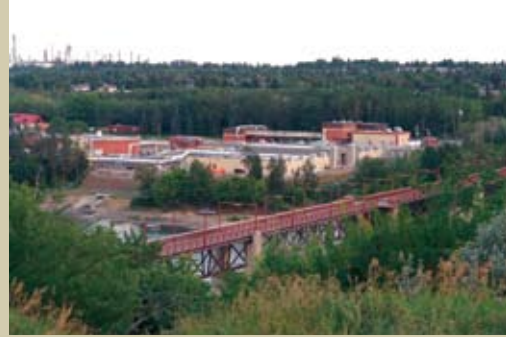
The City of Edmonton's Gold Bar Wastewater Treatment Plant used new material technology developed in the precast concrete industry for processing equipment in a recent expansion project. Photo courtesy of Tucker Photography.
