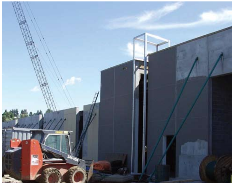
This view shows construction of the exterior walls. Photo courtesy of Lafarge Canada Inc.
