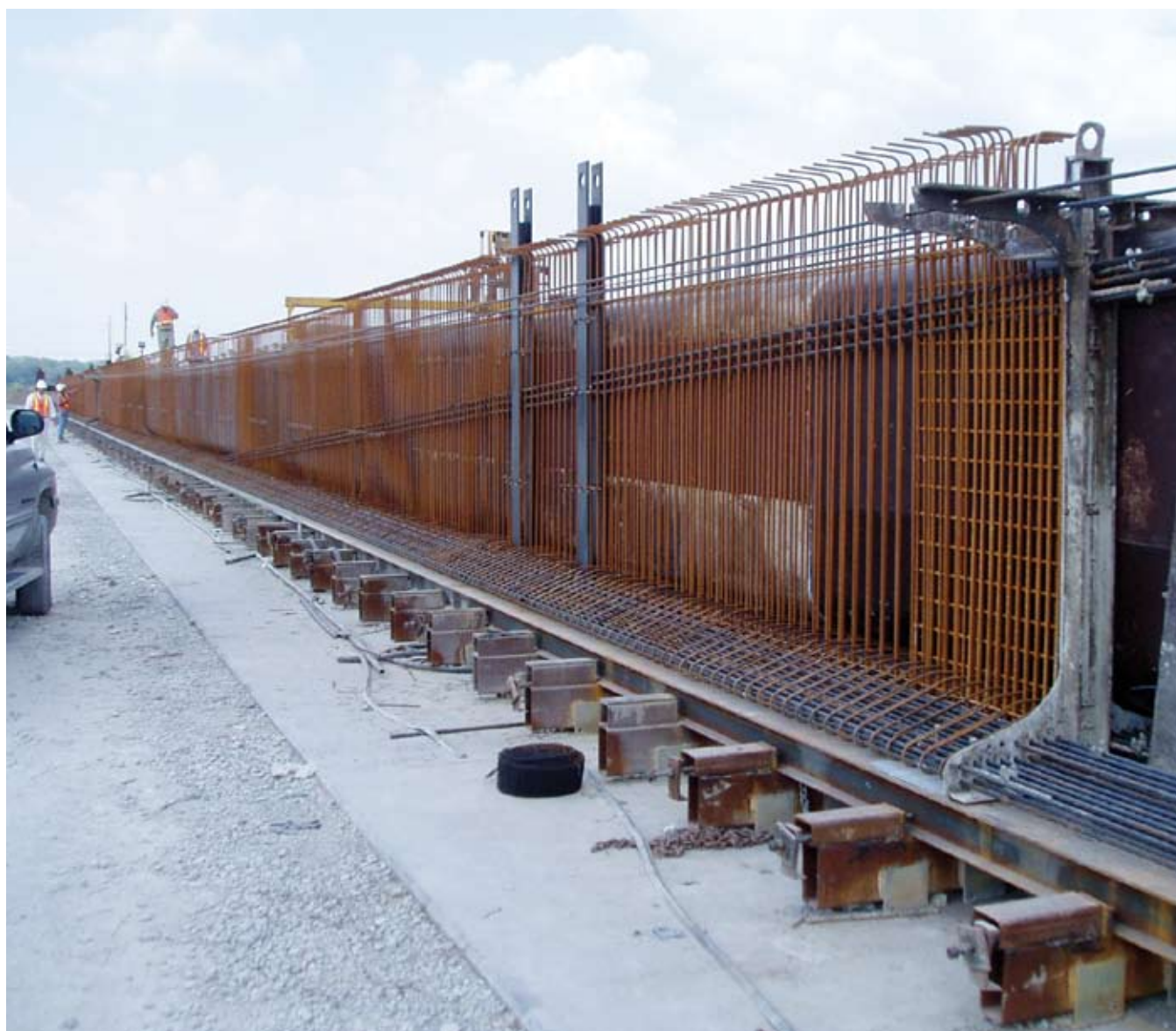
Fig. B8. Platte River East Bridge girder in Nebraska during fabrication.
